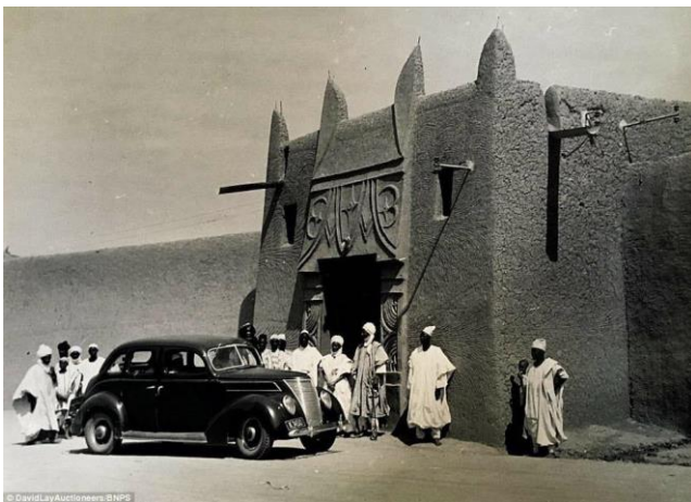
Figure 0.14 The 18th century Main (south) gate of Emir's Palace (ngconsulate, 2024)
