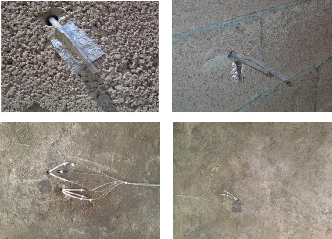
Figure 4.5. Replacement of thermocouple housing plastic tubes
