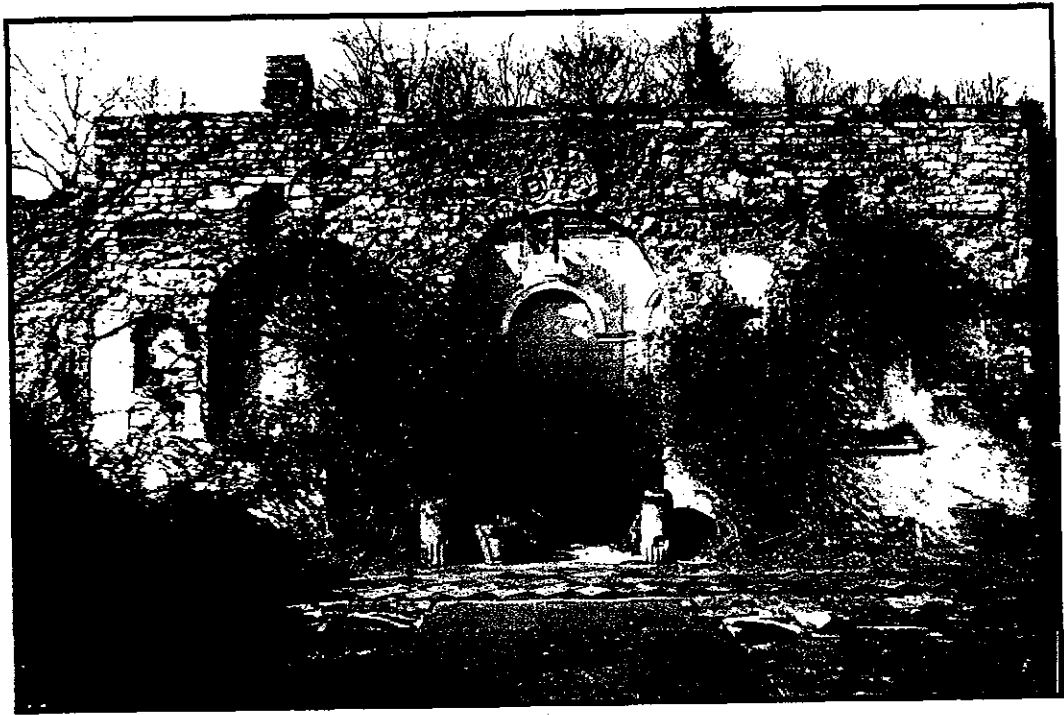
Figure 13. The Greenhouse south-facing on the west of the Hall
