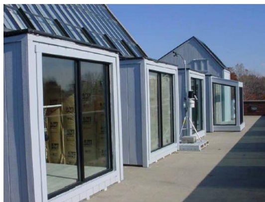
Figure2.3 South view of the five passive solar test-cells (from the left): Direct Gain (DG), Trombe-wall (TW), Water-wall (WW), Sunspace (SS), and Roofpond (RP). (Fernandez- Gonzalez A., 2007).
