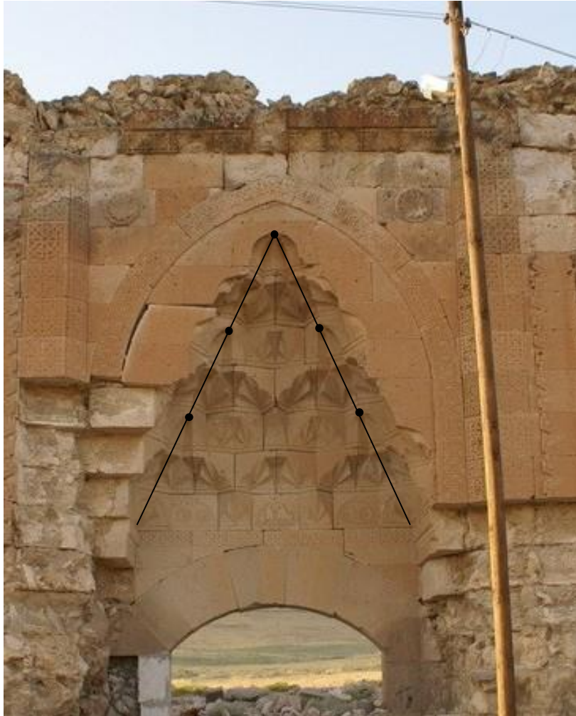
Figure 7 The first muqarnas portal in Anatolia, Alayhan Caravanserai. Lines representing diagonals and dots are geometric modules
