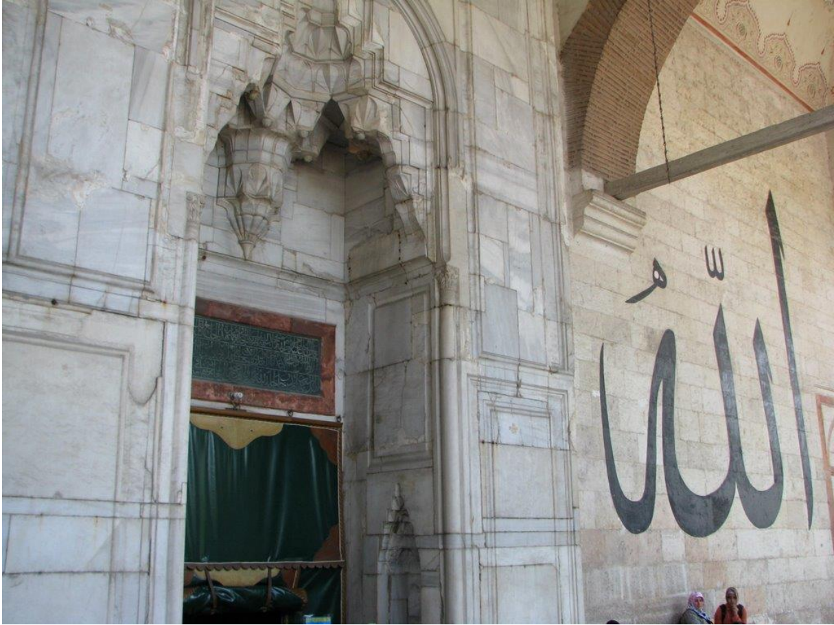
Figure 45 Edirne Old Mosque Portal.
