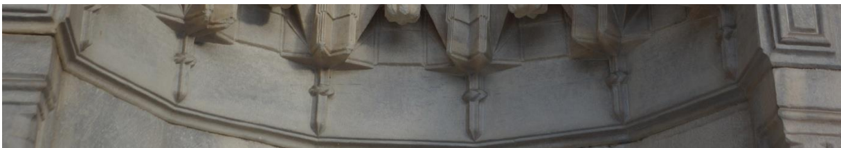
Figure 28 The last tier finishing with Kazayagis at Sultanahmed Mosque mihrab.
