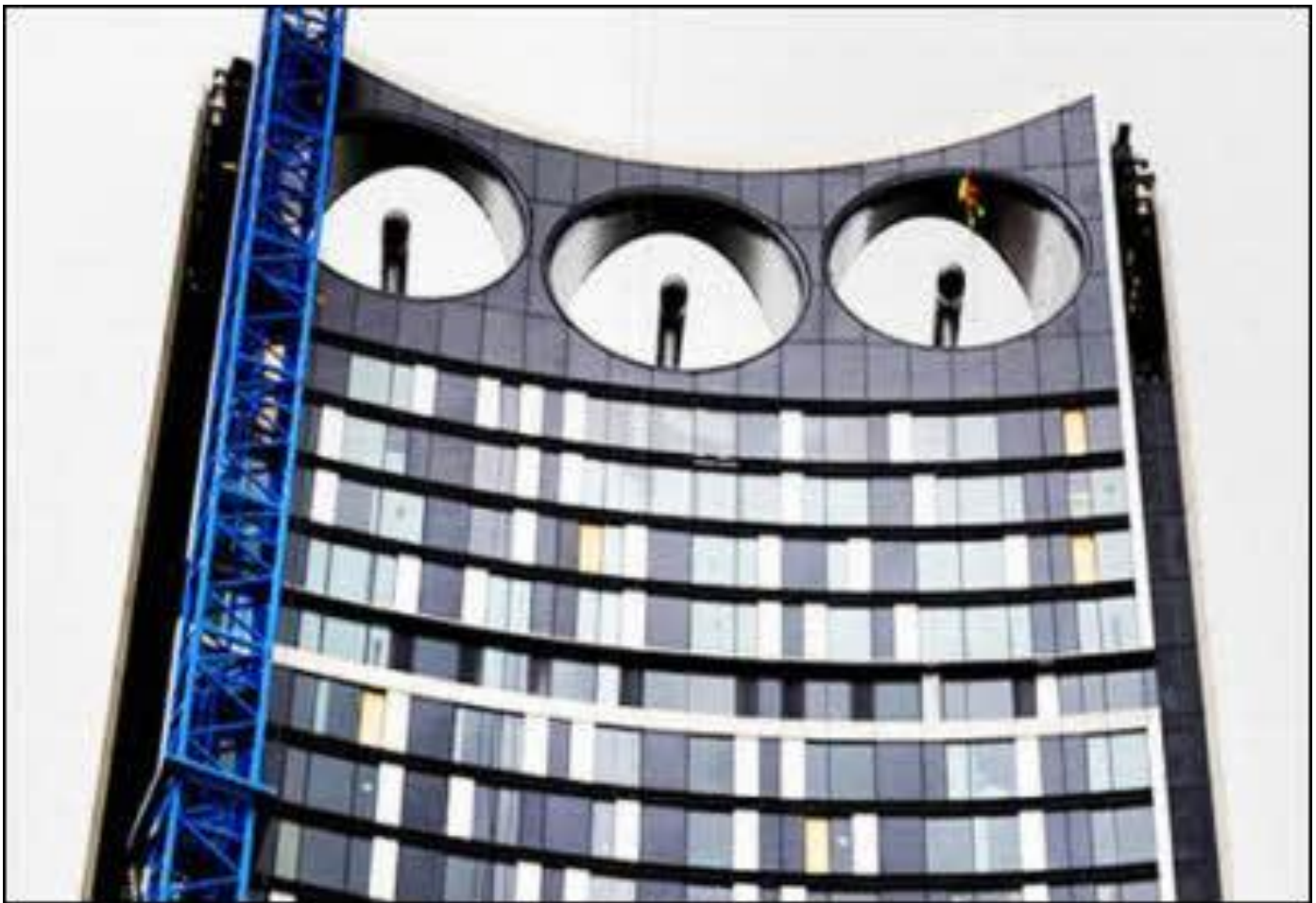
Figure 16 The $172 million Strata Tower in London harnesses wind energy with its three built-in turbines (URL 7)
