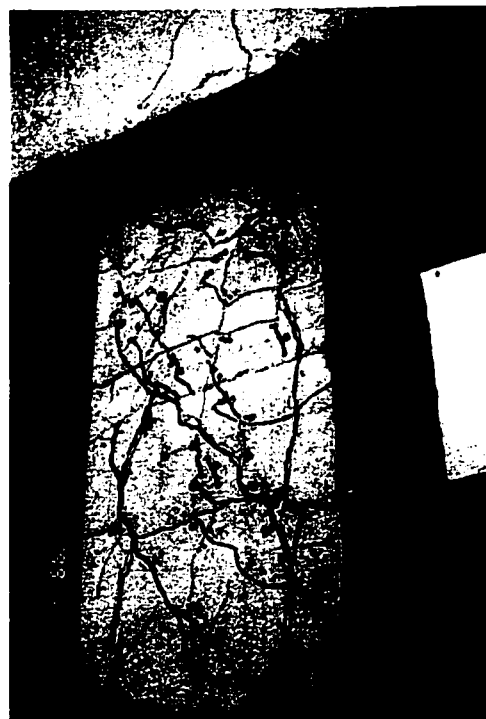
(b) upper portion of column(north-west)
