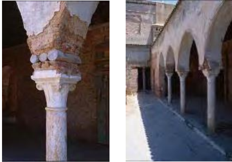
Figure 1.5. Historical structure, Medina [3]
