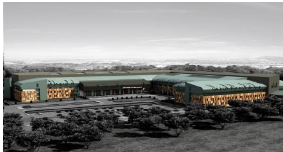
Figure 1.15. Van maternity hospital [14]
