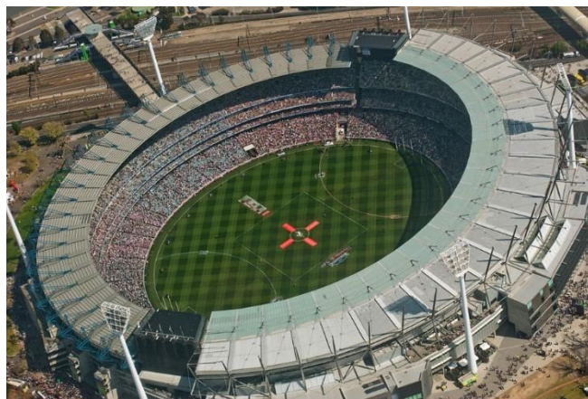
Figure 2.54 General view of the Melbourne Cricket Ground in 2010 (Sheko, 2010).
