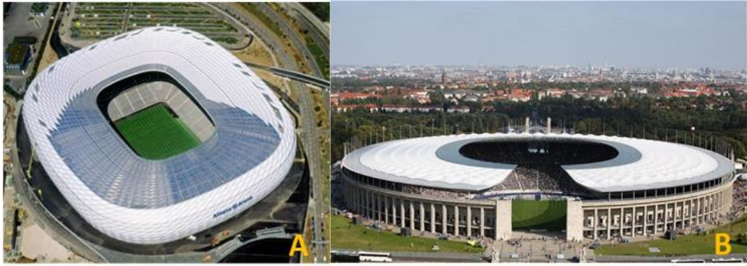
Figure 2.11 Examples of Cantilever roof structures. A: Cantilever roof structure of Allianz Arena, Munich, Germany. B: Cantilever roof structure of Berlin Olympic Stadium, Berlin, Germany (Allianz Arena, 2015; Olympiastadion, 2015).
