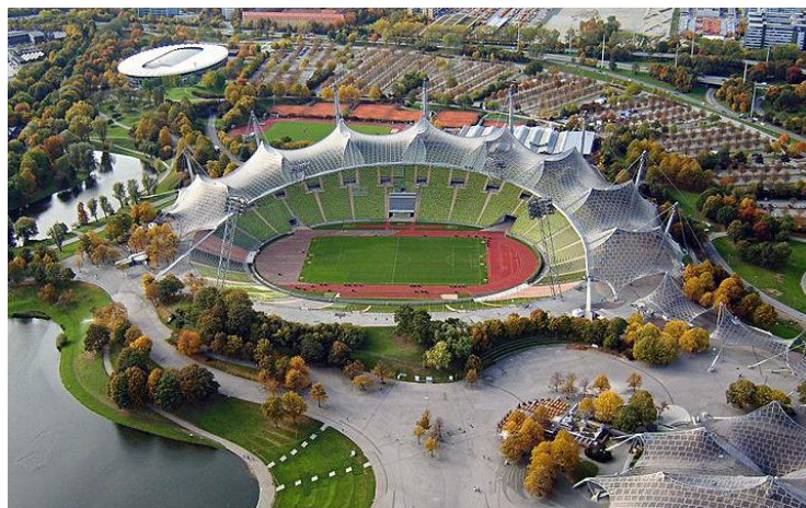
Figure 2.15 Cable net roof over Munich Olympic Stadium 1972, Munich, Germany (Mojtahedi, 2008).
