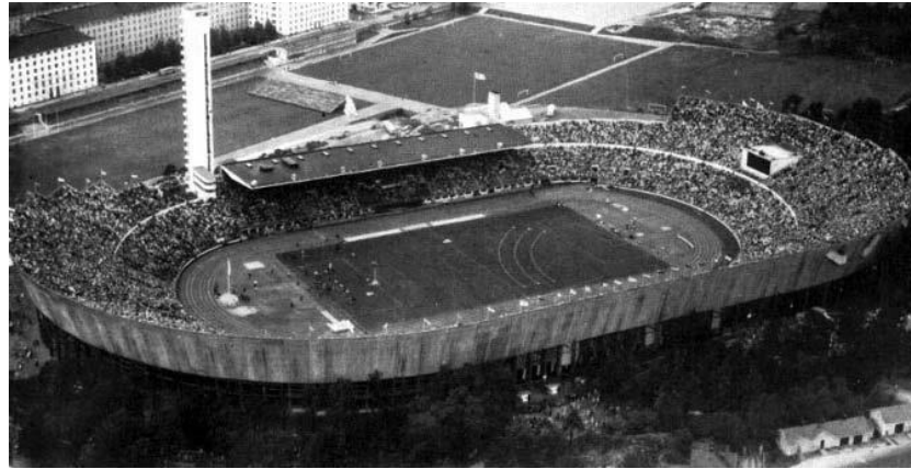
Figure 2.51 General view of Olympia-stadion Helsinki in 1952 (OCOH, 1955, p.44).
