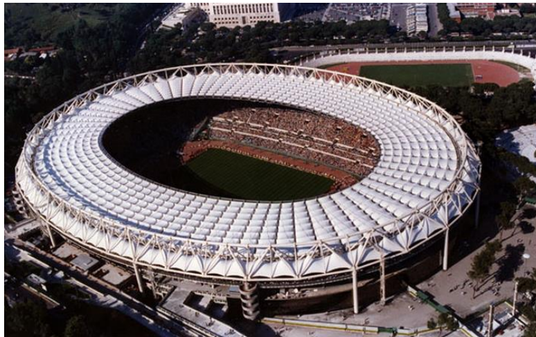
Figure 2.13 Compression Tension ring structure over Rome Olympic stadium, Rome, Italy (Zennit, 2015).
