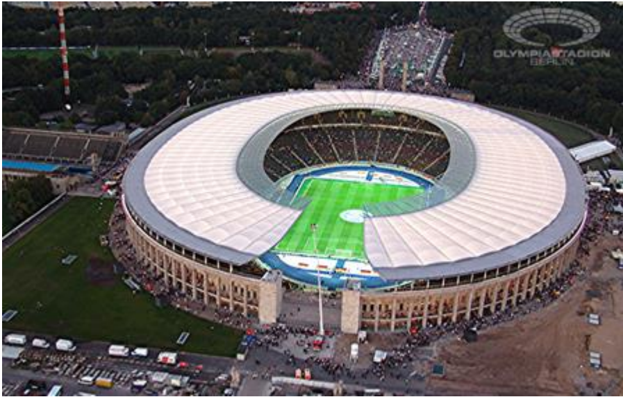
Figure 2.48 General View of Olympia stadion Berlin after erection of continues roof in 2000 (Busam, n.d.).
