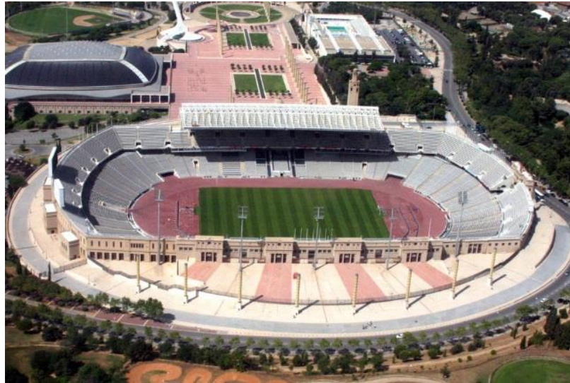
Figure 2.68 General view of the Barcelona Olympic Stadium in 1992 (COOB'92, 1992, p.162).
