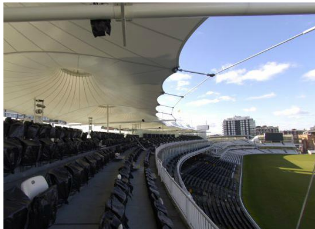
Figure 2.16 The membrane roof structure over the Mound Stand at Lord's Cricket Ground, London, England (Hogg, 2006).
