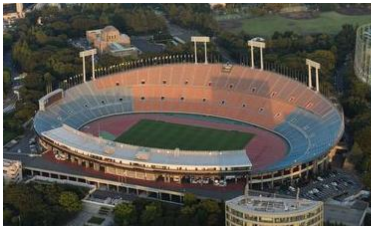
Figure 2.58 General view of Tokyo National stadium in 2013 (Tomura, 2013).
