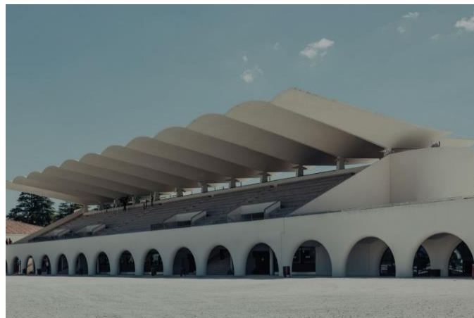
Figure 2.12 Concrete shell structure over the grandstand of Zarzuela Racecourse, Madrid, Spain (Michavila, n.d).
