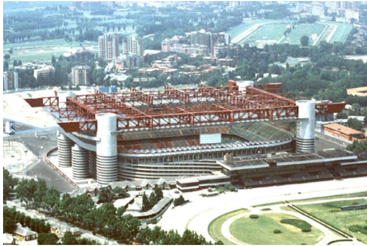
Figure 2.18 Space frame roof over the San Siro stadium, Milan, Italy (Vittorio, 2014).
