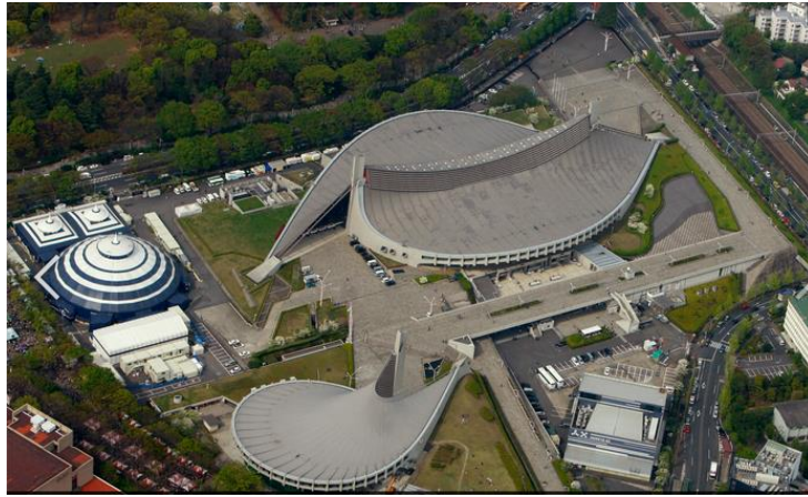
Figure 2.14 Catenary Cable Structures built for Twin gymnasias designed by Kenzo Tange for the 1964 Olympic Games, Tokyo, Japan (Whiting, 2014).
