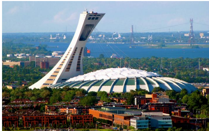
Figure 2.64 General view of Montreal Olympic Stadium in 2009 (Julius, 2009).
