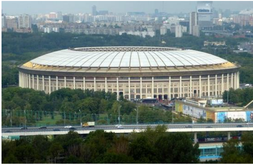
Figure 2.66 General view of the Luzhniki stadium in 2010 (Muehlbradt, 2010).
