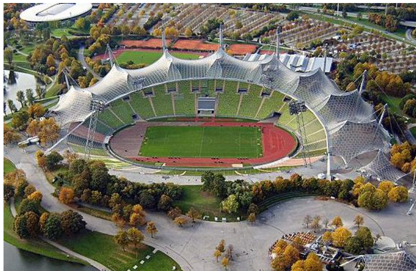
Figure 2.62 Cable net roof structure over the Munich Olympic Stadium in 1972 (Mojtahedi, 2008).
