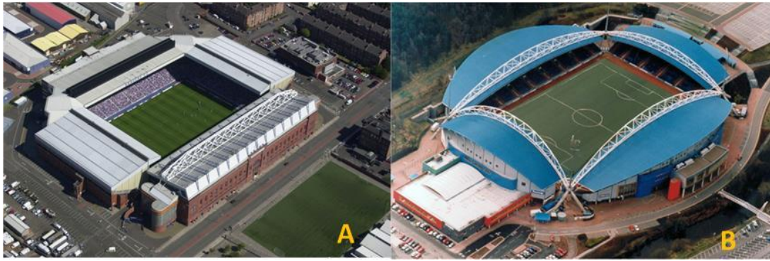
Figure 2.10 Examples of Goal Post structures. A: Goal post roof structure of Ibrox Stadium, Glasgow, Scotland. B: Goal post roof structure of Galpharm stadium, Huddersfield, United Kingdom. (Rangers, 2015; johnsmithsstadium, 2015).
