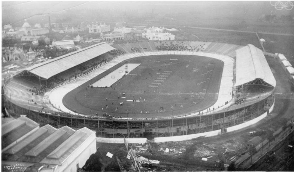
Figure 2.9 Post and Beam roof structures cover the East and West stands of White City Stadium, London, England (Olympic Games, 1908).
