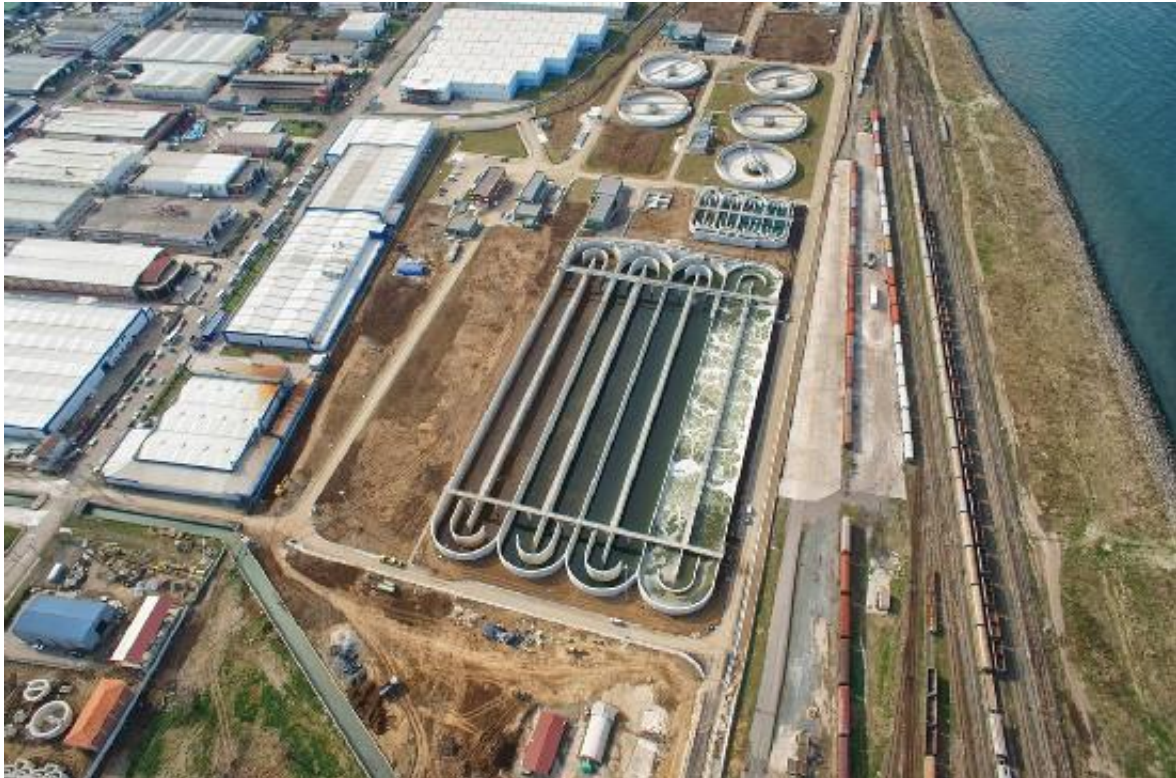
Figure 3.2 : Samsun Doğu Advanced Biological Wastewater Treatment Plant.
