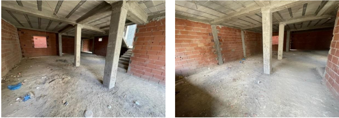
Figure 128. Interior views of new open-plan villas, ‘Villas Benbellat-Tazoult’ (Source: Images captured by the author, Batna, February 2024)
