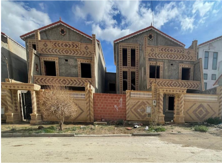
Figure 38. The newest villas under construction in ‘Villas Benbellat’. (Source: Image captured by the author, Batna, February 2024)
