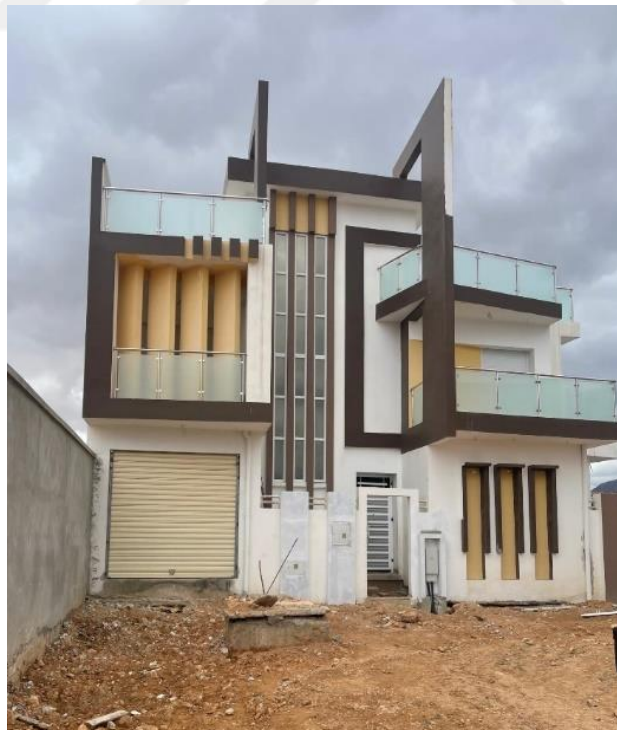
Figure 74. Exterior view of a typical villa in 'Marwa Residence'. (Source: Author's photo, February 2024)
