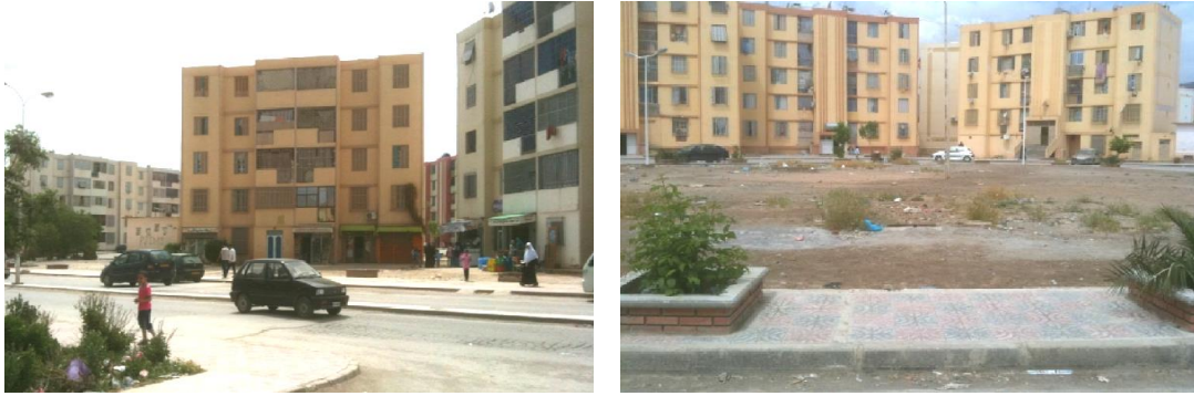
Figure 26. A ZHUN project, 1020 housing unit neighbourhood, Batna. (Source: Guerarra, Revalorization of New Urban Housing Areas, 144)
