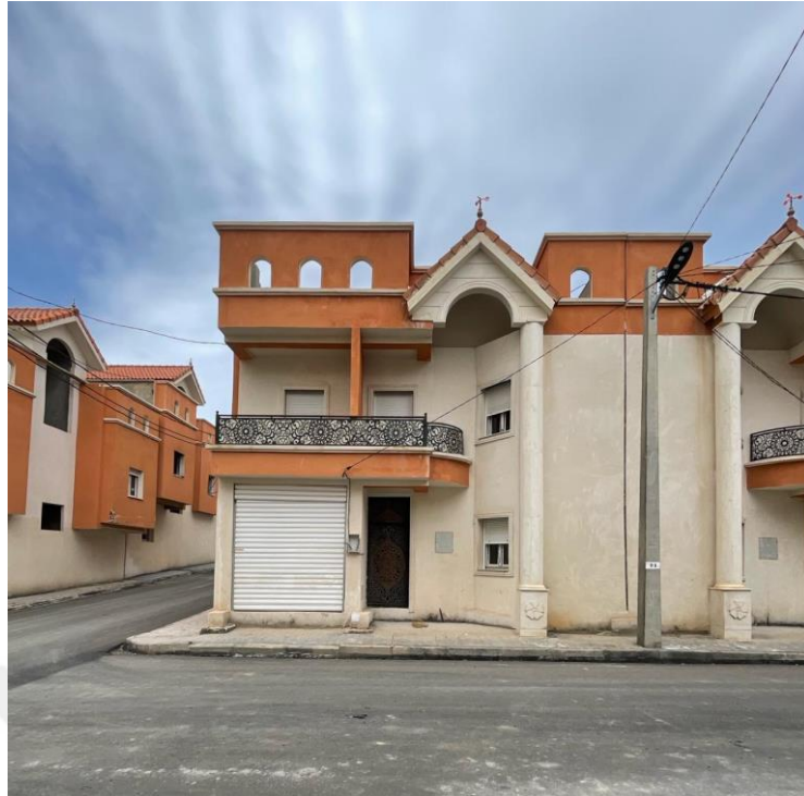
Figure 67. Main façade of villa type 01 in ‘648 housing units’. (Source: Image captured by the author, Batna, February 2024)
