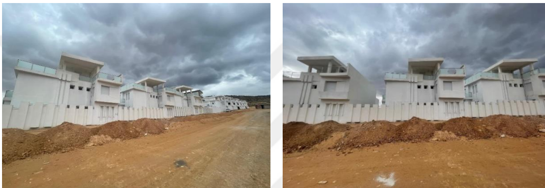
Figure 76. Exterior view on ‘Marwa Residence’. (Source: Image captured by the author, Batna, February 2024)
