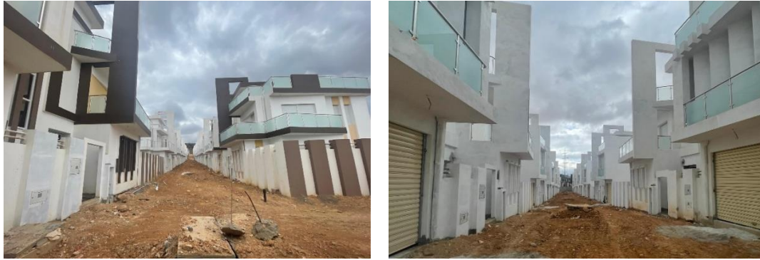
Figure 75. Typical villa row, under construction, ‘Marwa Residence’. (Source: Images captured by the author, Batna, February 2024)
