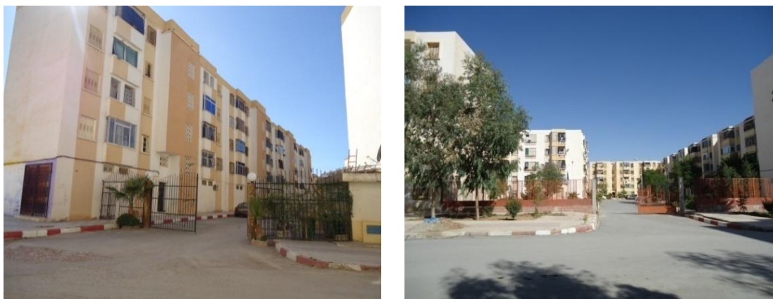
Figure 16. Metal Fences in Mass Housing, Hamla Neighbourhood, Batna. (Source: Bendib, "Residential Self-Enclosure," 3-4)
