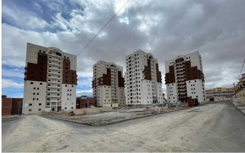
Figure 60. View of apartment blocks in the ‘648 housing units’. (Source: Image captured by the author, Batna, February 2024)
