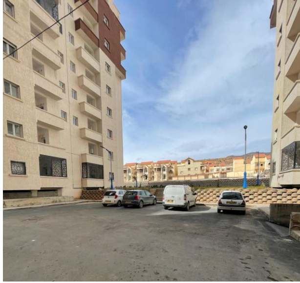
Figure 62. View of the first parking area in '648 housing units'. (Source: Author's image, February 2024)
