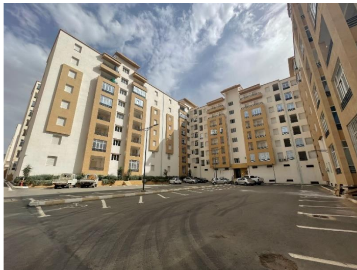
Figure 45. View of the parking area within the GC ‘Résidence Bezzala’. (Source: Image captured by the author, Batna, February 2024)
