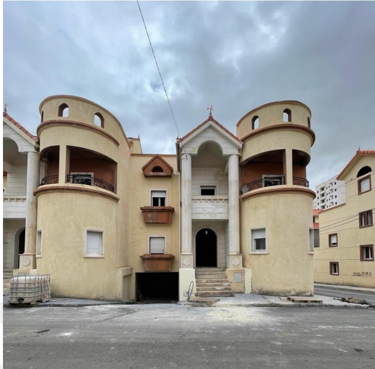
Figure 69. Main façade of villa type 02 in ‘648 housing units’. (Source: Image captured by the author, Batna, February 2024)
