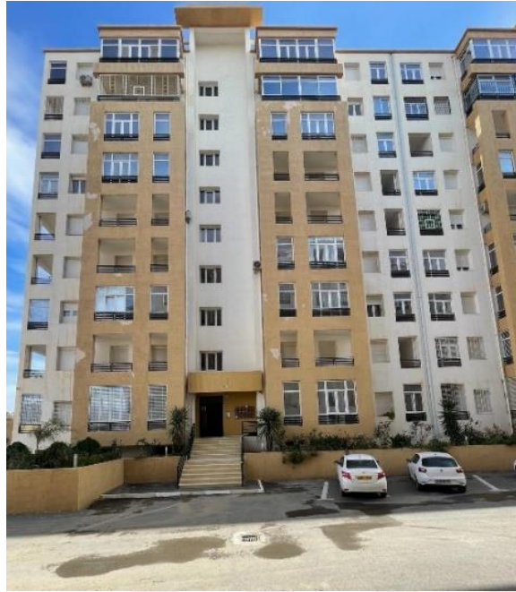
Figure 78. Typical apartment block, front view, 'Résidence Bezzala'. (Source: Image captured by the author, Batna, February 2024)
