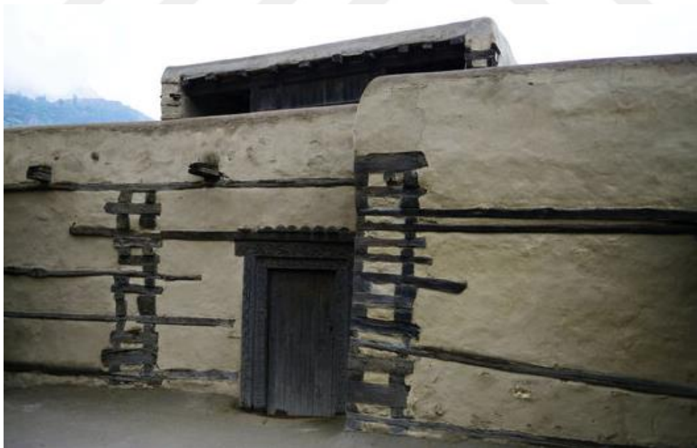
Figure 5.21 A Blow-up of the adopted Preservation Technique in Baltit Fort. (Photograph taken by Author)
