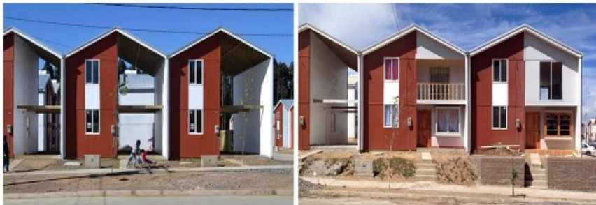
Figure 2.4. Temporary housing as a core shelter example. a) primary building provides infrastructure and basic spatial needs b) secondary building as a permanent house
