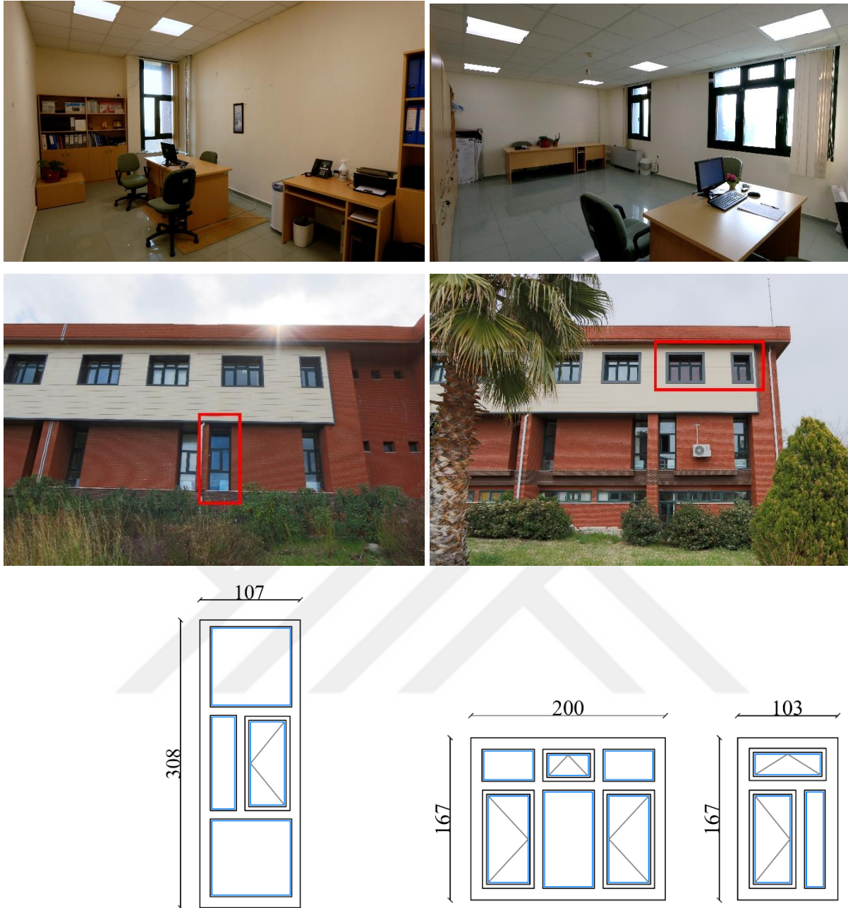
Figure 3.2. Interior view, exterior view and window dimensions of north-facing (left) and south-facing (right) rooms
