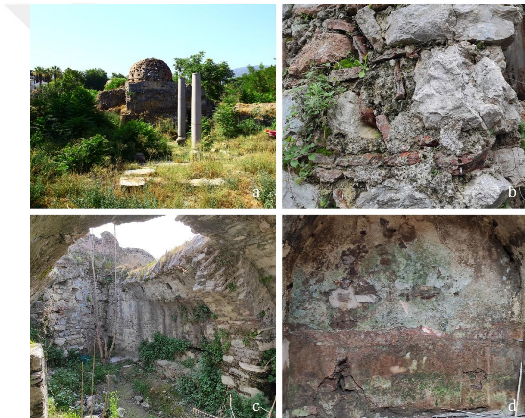
Figure 3. 8. Structure failures and material deterioration (probably due to weather conditions, rainwater penetration, rising damp, lack of maintenance, seismic forces, or vandalism): Plant growth (a), Joint discharge (b), Discoloration, (c), Microbiological colonization (d)
