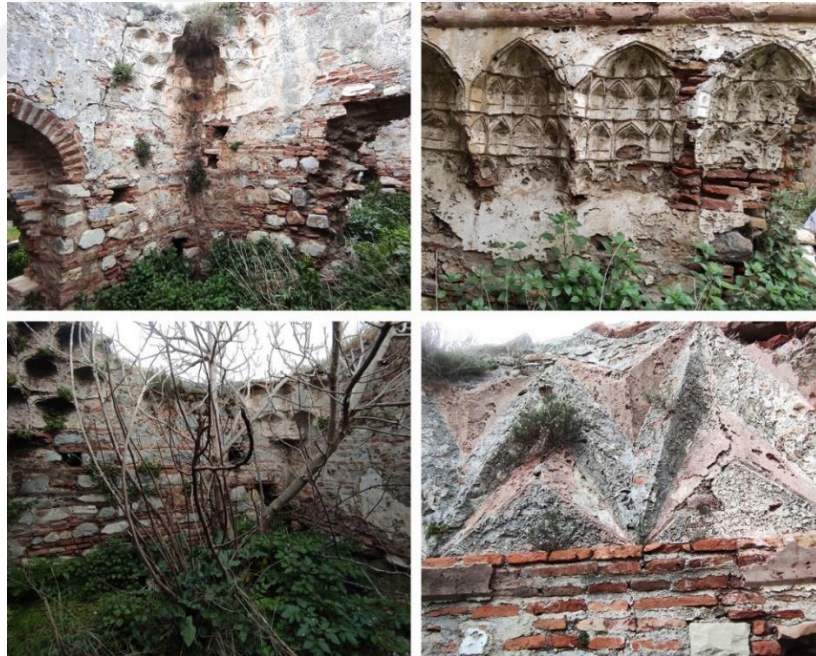
Figure 3. 11. Structure failures and material deterioration of Kale Altı Bath: Structure failures and material deterioration (probably due to weather conditions, rainwater penetration, rising damp, lack of maintenance, seismic forces, or vandalism): Joint discharge (a), Discoloration (b), Plant growth (c), Microbiological colonization (d)
