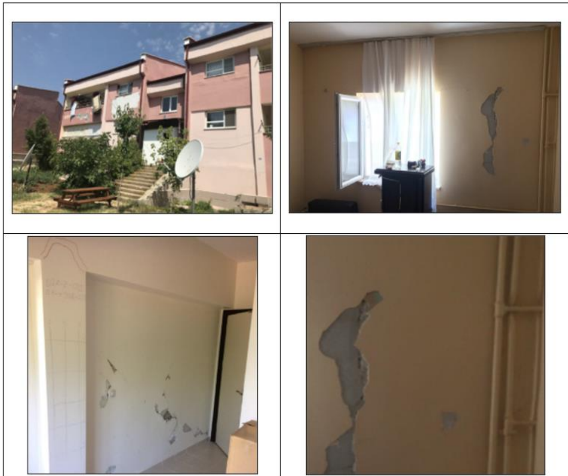
Figure 6.3. Photographs of Building #2
