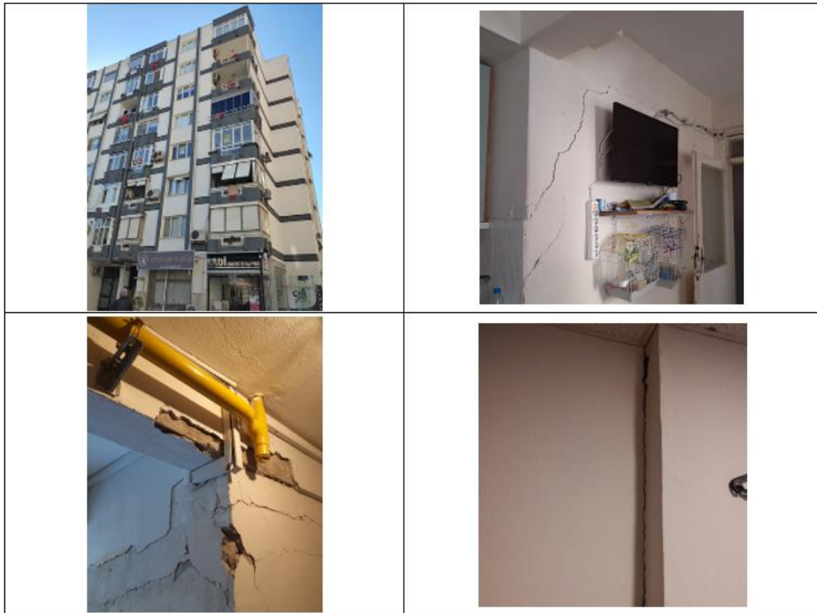
Figure 6.23. Photographs of Building #12
