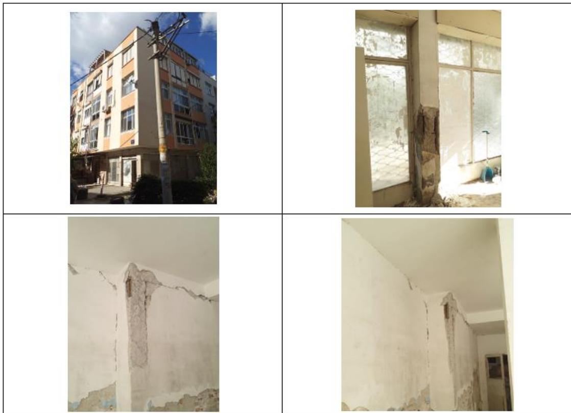
Figure 6.21. Photographs of Building #11
