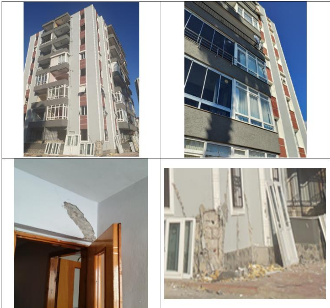
Figure 6.13. Photographs of Building #7
