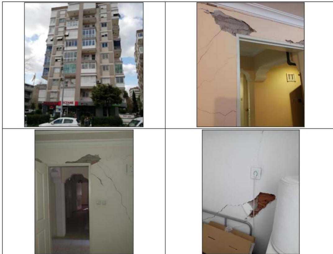
Figure 6.29. Photographs of Building #15
