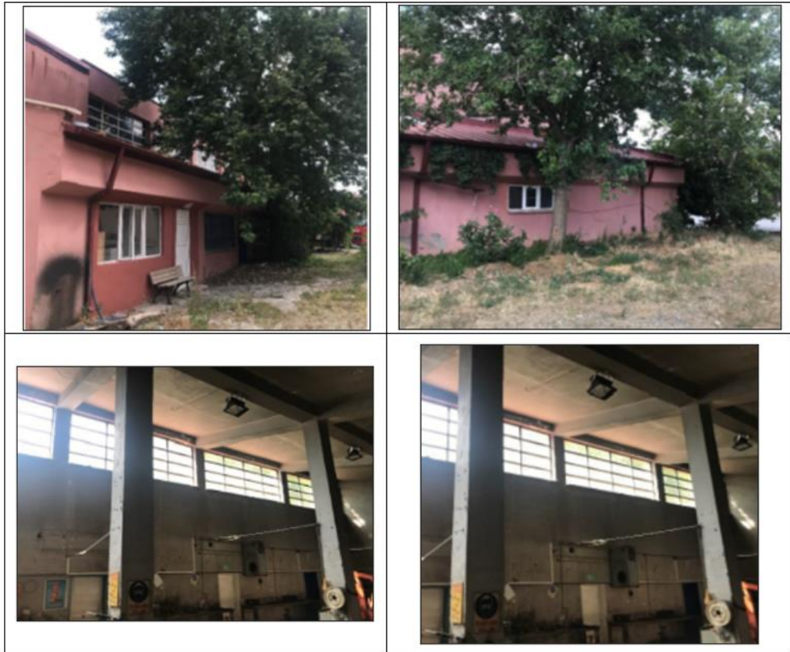
Figure 6.7. Photographs of Building #4
