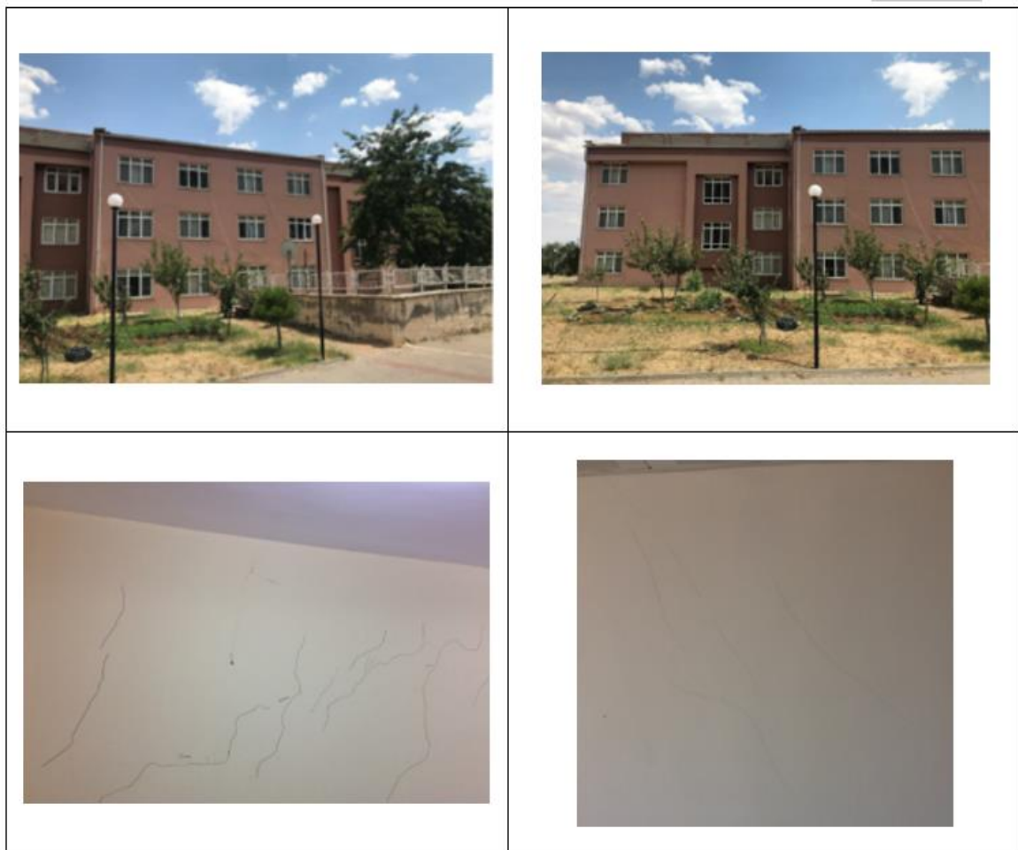
Figure 6.11. Photographs of Building #6
