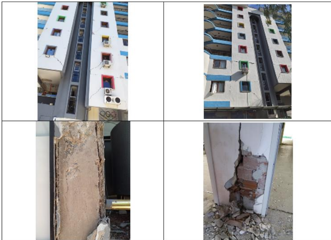
Figure 6.25. Photographs of Building #13
