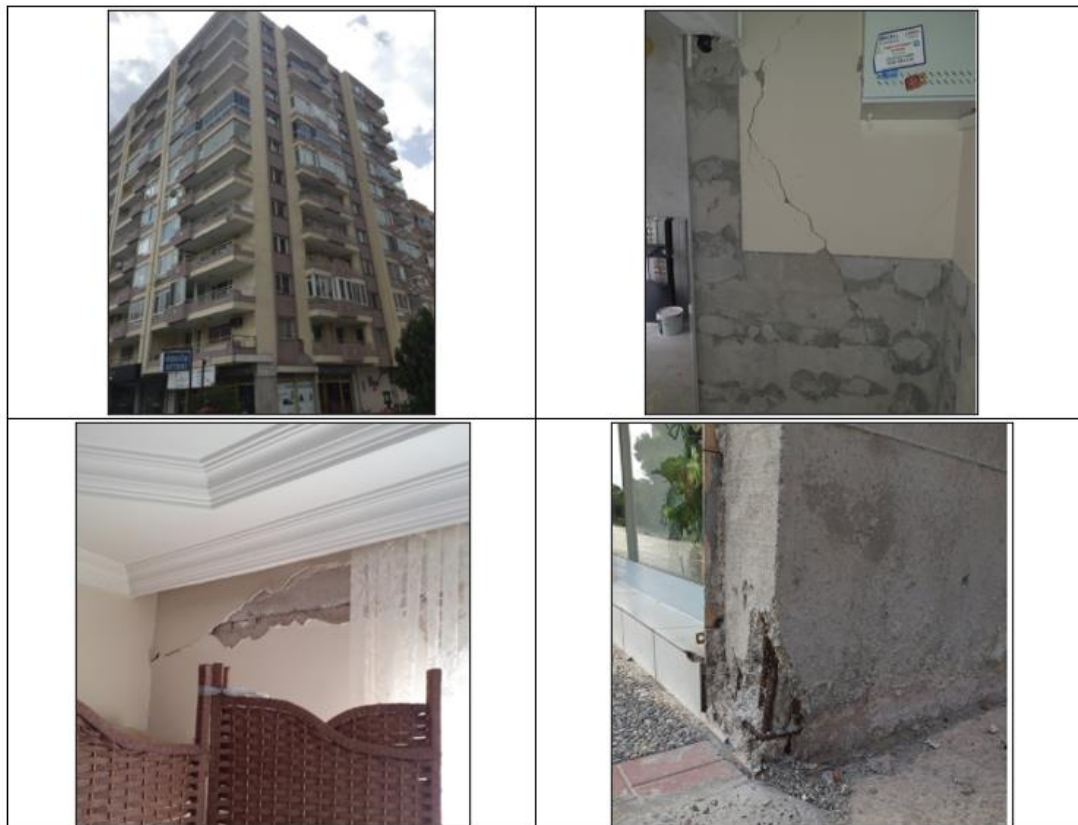
Figure 6.27. Photographs of Building #14
