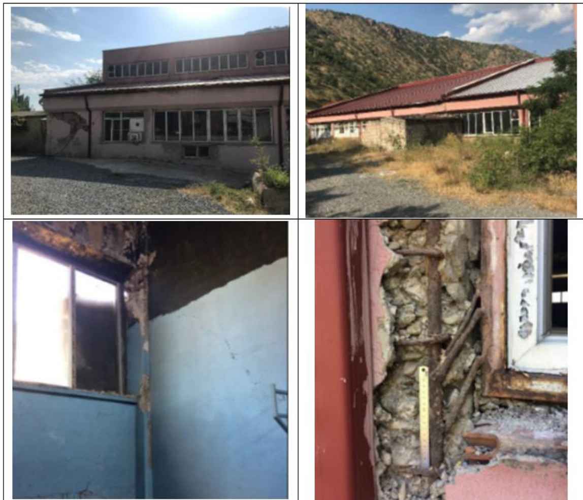
Figure 6.9. Photographs of Building #5
