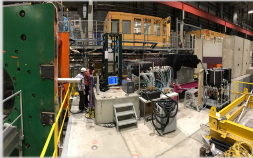
Figure 4.2. Installation of the HGCAL and AHCAL prototype at PPE172 zone.
