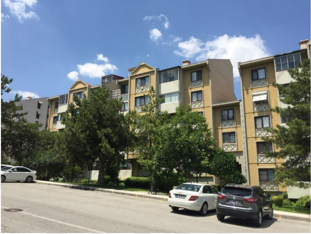
Figure 4.42. Konutkent II, Type C Blocks, June 2018 (Photograph by E. Ünver)
