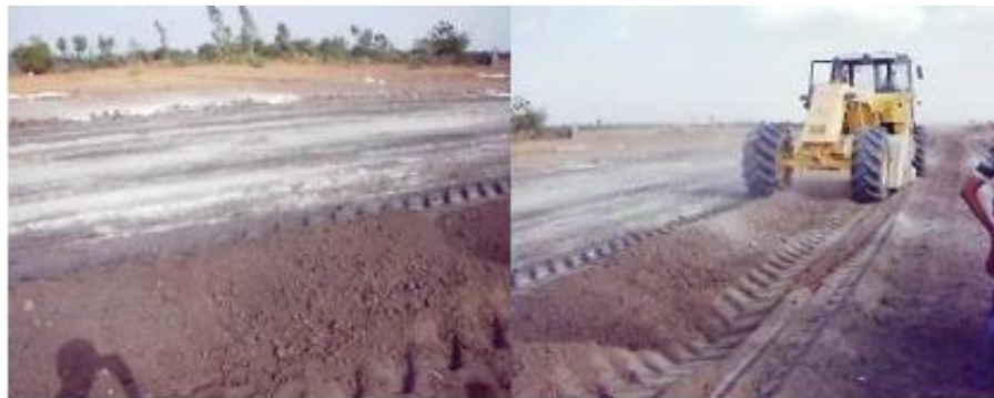
Figure 2.11 : Laying of lime/fly ash and onsite mixing machine.
