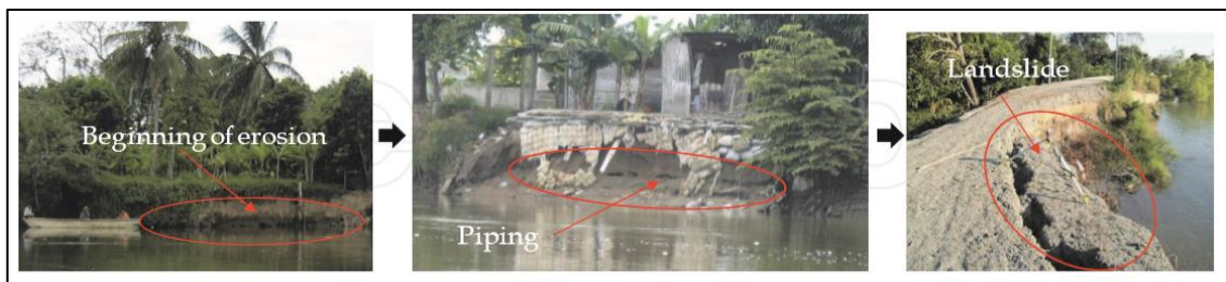
Figure 3.14 Evidences of instability in river embankments caused by erosion (Source: Jeanmonod and Rebecca 2018)
