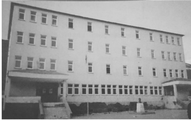
Figure 3.5 The photo of the 4-story existing school building
