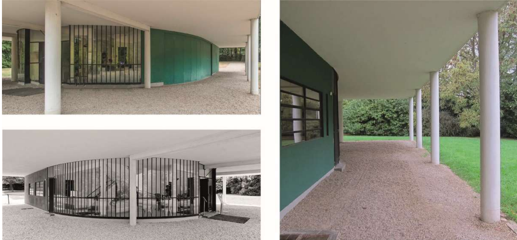
Figure 139 Membrane facade of the ground floor.
