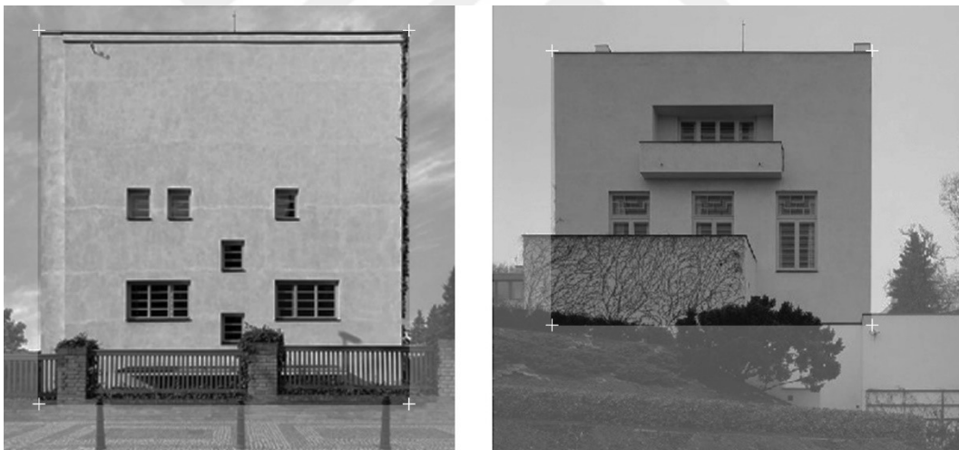
Figure 125 Image on the left: Villa Müller's Southwest Facade. Source: 20th Century Design, instagram.com/b22_design . Image on the right, Northeast Facade. Source: Architectuul, https://architectuul.com/architecture/villa-muller (Edited by the Author).
