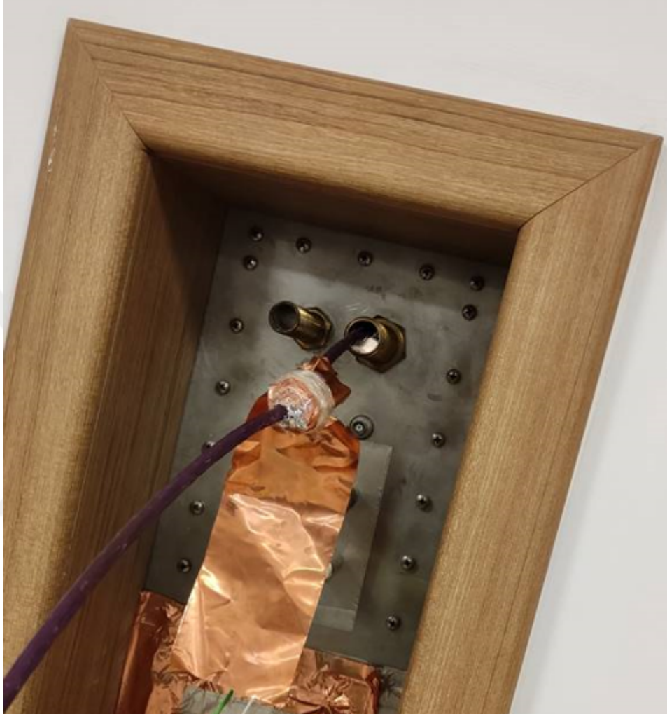
Figure 3.4: Unifying LVDS RF pulse information carrier CAT7 ethernet cable's shield with the main MRI scanner room's Faraday cage
