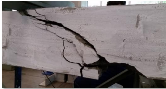
Figure 2.4 Shear failure of deep beams in laboratory experiment by Tuladhar, 2014
