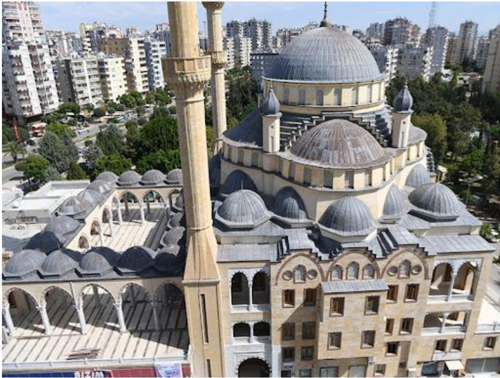
Figure 4.4. Ramazanoğlu Mosque aerial viewpoint (source: http://www.cukurova.gov.tr/ramazanoglu-cami )
