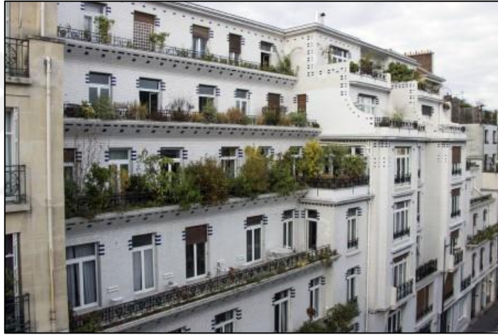
Şekil 9. Rue Vavin binası ( https://blog.parisinsights.com/henri-sauvages-stepped-terrace-apartment-building/ )
