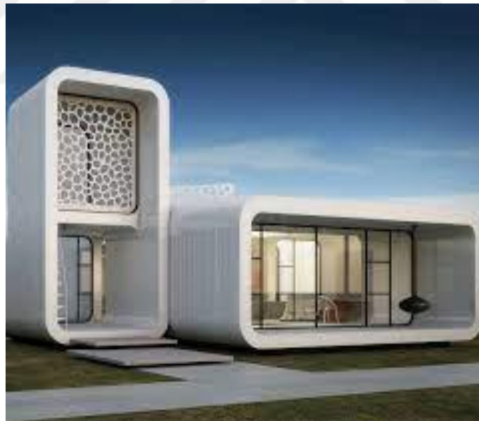
Figure 2.2. Building in the UAE built using 3D printing [30].
