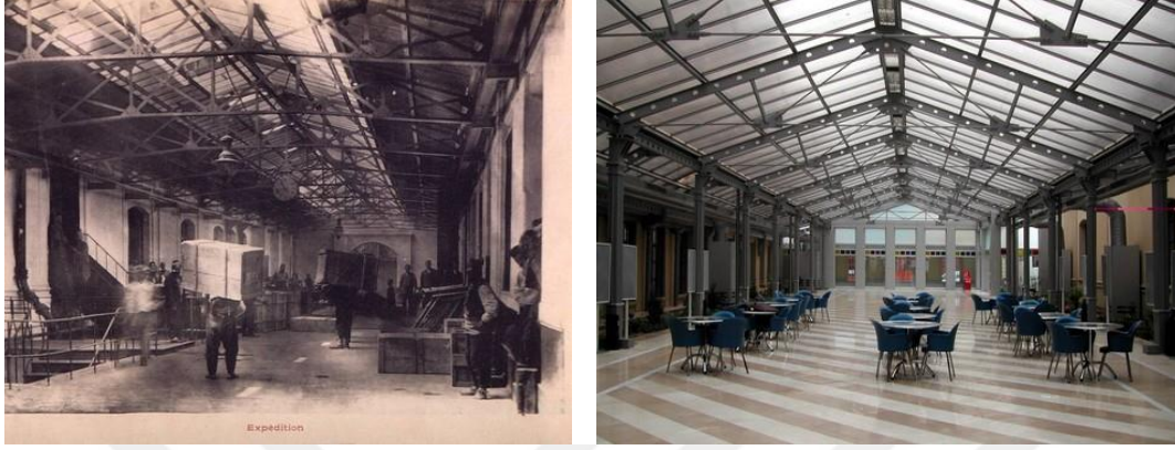
Figure 2.9: Cibali Tobacco Factory 1884-1995 and Kadir Has University Cibali Campus currently in use.
