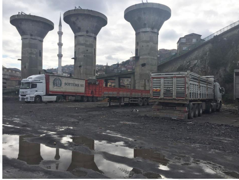
Figure 4.27: What is left from Zonguldak Coal Washery Area, and in the background the city silhouette, December, 2017, (Photograph by İ. Çörek)
