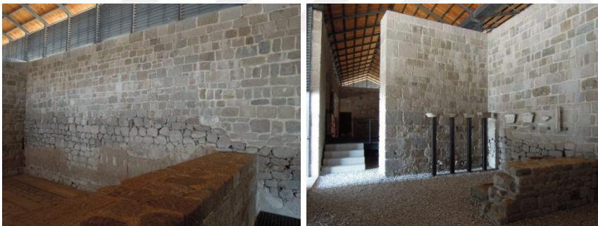
Figure 4.16 New walls on top of original walls (left), and exhibited fragments (right), Pergamon (the author 2011)
