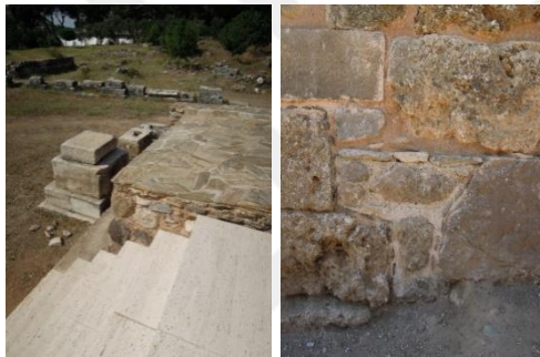
Figure 3.98 The steps and the perimeter wall (left) (the author 2015); (right) infill in the perimeter wall (right) (the author 2011)
