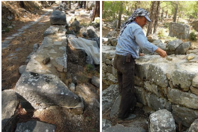
Figure 4.7 Mortar capping, Priene (the author 2011)
