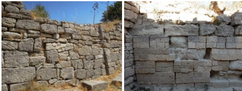
Figure 4.11 Examples of the infill technique, Troy (the author 2011)
