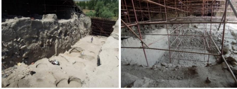
Figure 3.72 Shelter covering an excavated trench (the author 2015)
