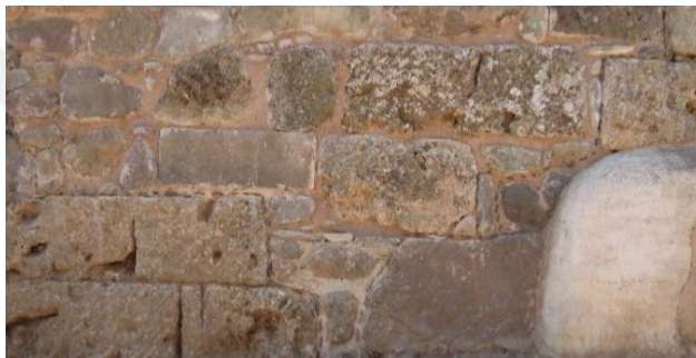
Figure 4.10 Use of broken slates to distinguish infill, Sardis (the author 2011)
