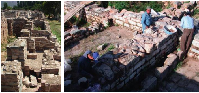
Figure 4.6 Mortar capping, Aphrodisias (Proudfoot & Severson 2010:203–204)
