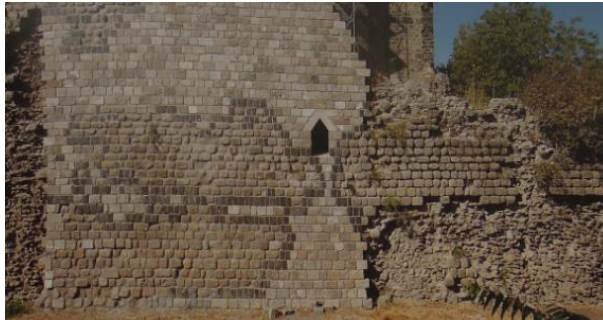
Figure 4.9 Use of basalt to distinguish infill, Pergamon (Bachmann 2014b:95)
