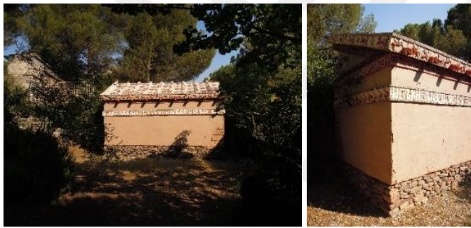
Figure 3.96 Reconstructed Lydian building (the author 2015)
