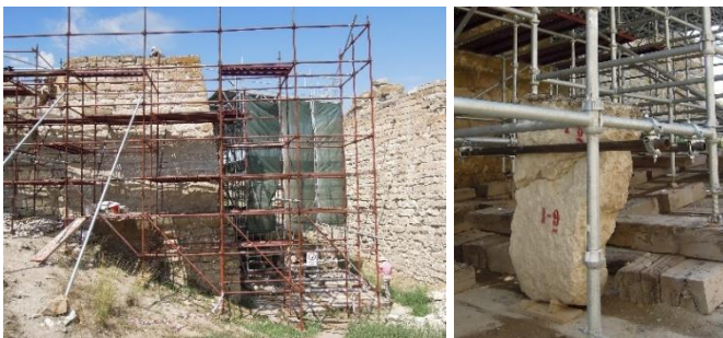
Figure 3.90 The scaffolding erected in 2014 for the new interventions at the monumental gateway (left) (the author 2015); dismantled and repaired stone from the gateway (right) (the author 2015)
