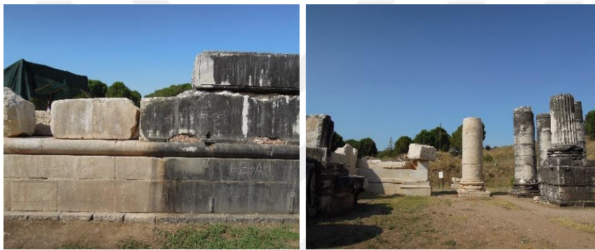
Figure 4.12 Biocide applied surfaces vs ‘uncleaned’ surfaces, Sardis (the author 2015)
