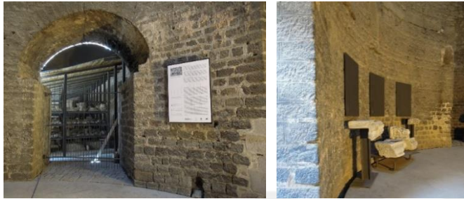
Figure 3.34 Inside of the tower (the author 2011)
