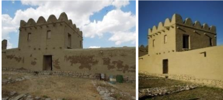
Figure 4.17 Maintenance of the city wall (before and after; same season), Hattusha (the author 2015)
