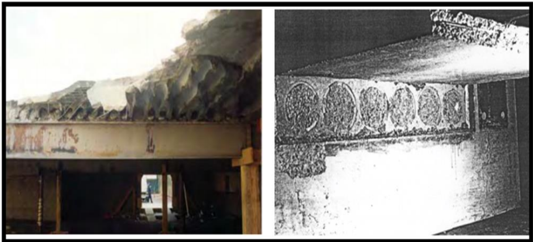
Figure 1.1 Failure of hollow-core in the 1994 Northridge earthquake [5] and experimental test [6]
