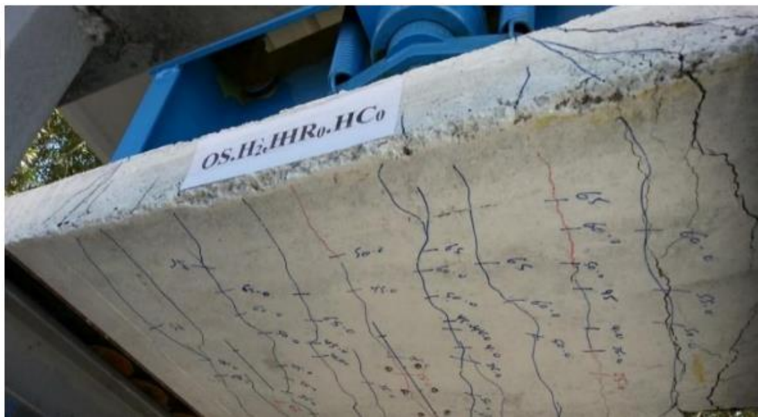
Figure 2.7 Mode of failure and cracks pattern of HCS [12]
