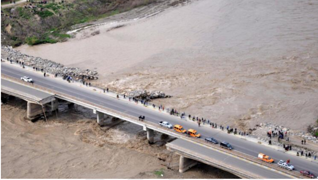
Figure 1.1 Çaycuma bridge after the collapse (Ercan & Gündoğan, 2015)
