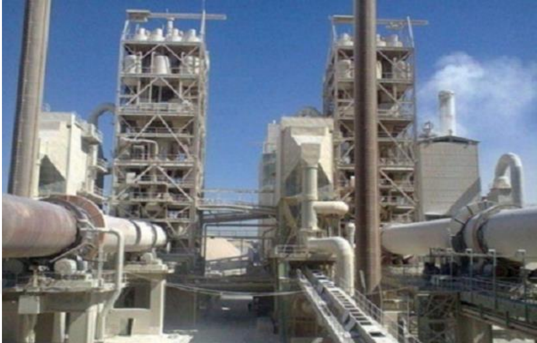
Figure 1.1. Fallujah White Cement Plant.
