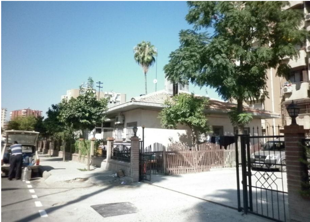
FIGURE 6.2.-6: State Railroad Workers Housing, 2012 (Author's Archive)
