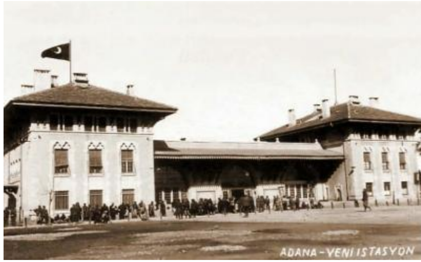
FIGURE 5.3.-1: Adana New Station Built 1912 (www.wowturkey.com)
