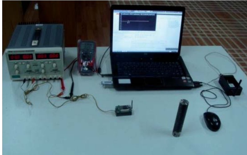
Figure 4.6.b A DC power supply provides the power of the sensor
