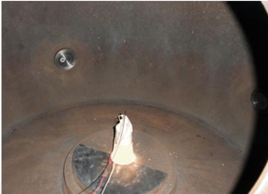
Figure 3-8 Positioned Charge Assembly with the Base Plate
