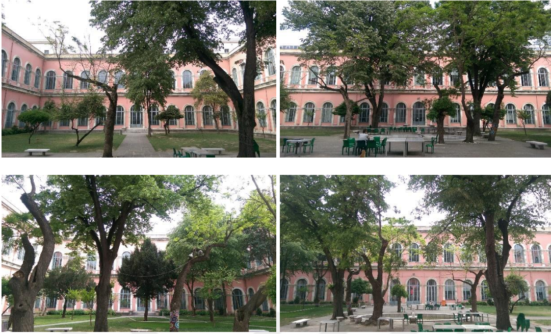
Figure 4.4 : Façades looking at courtyard.
