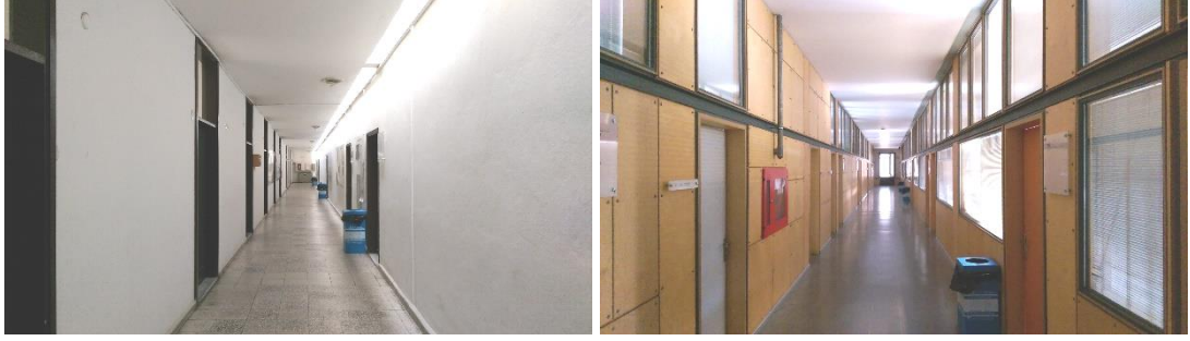
Figure 4.7 : Finishing differences on the roof floor.
