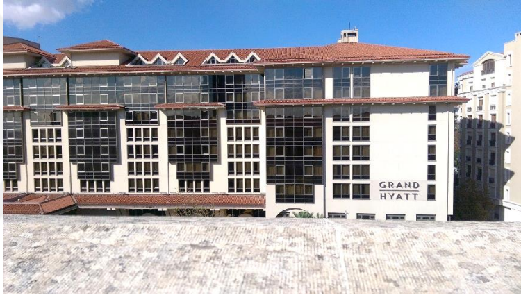
Figure 4.19 : View from the studio Çatı 2. Students can partially see the immediate surrounding of the building.
