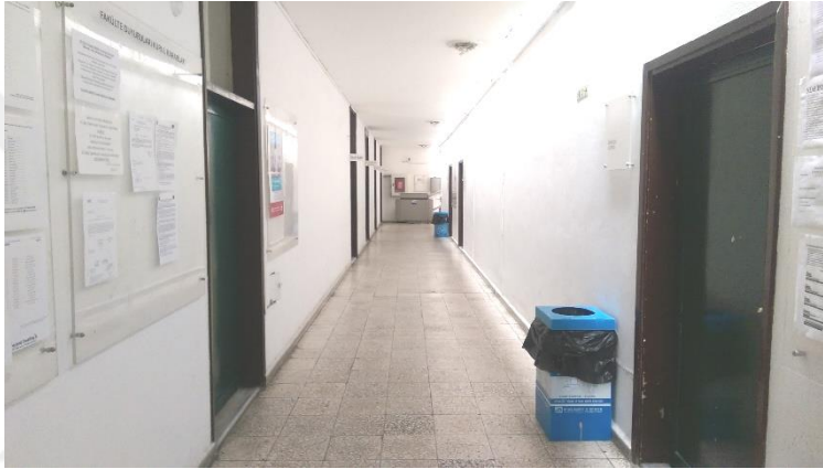
Figure 4.17 : View from in front of Registrars' Office. Students cannot see outside from this point.
