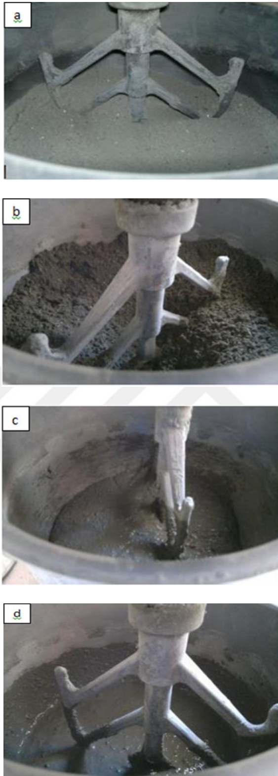
Figure 3.2 Mixing of UHPFRC, (a) dry mix, (b) water addition, (c) superplasticizer addition with low speed, (d) superplasticizer addition with high speed
