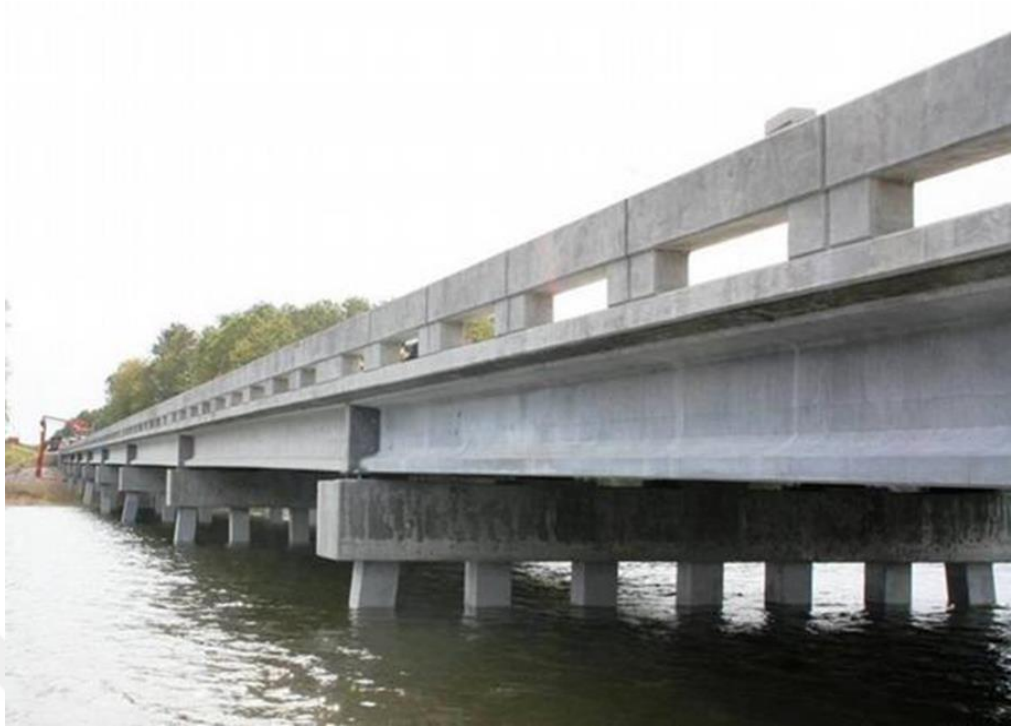
Figure 2.2- Cat Point Creek Bridge, Virginia, USA (Graybeal, 2009)
