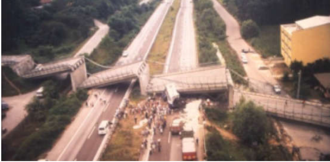
Figure 2.13: Arifiye Overpass (Erdik, 2001)
