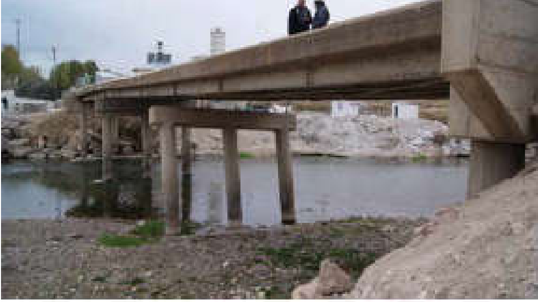
Figure 2.10: Photo of a Bridge after Van Earthquake that was damaged due to a flood few years before (23 Ekim 2011 Mw 7,2 Van Depremi Sismik ve Yapısal Hasara İlişkin Saha Gözlemleri, 2011)
