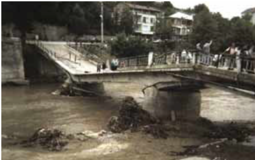
Figure 1.5. Damaged view of the bridge at Devrek due to scour (Yanmaz, 2002)
