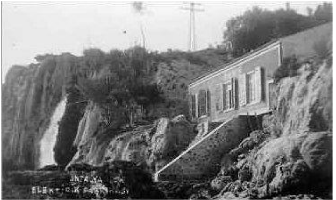
Figure 34 Energy Power Plant (source: Antalya KUDEB)
