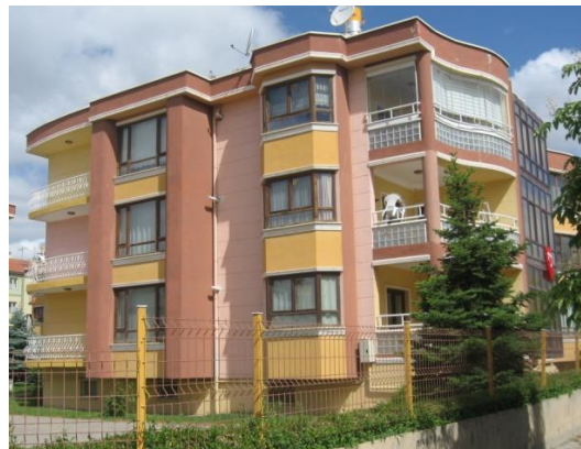
Figure 4.29 Examples of RC buildings from Erzincan; (a) shear wall RC building (RW) (b) frame RC building (RF) (c) dual RC building (RH)
