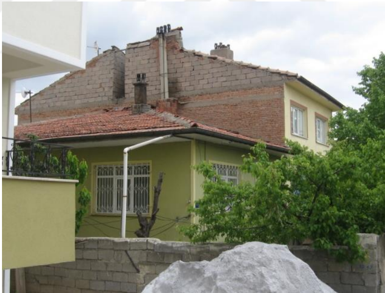
Figure 4.30 Examples of masonry buildings from Erzincan with varying material and construction quality
