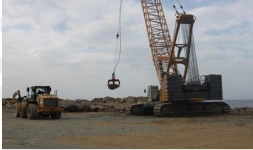
Figure 4.45 Arrangement of rockfill with Crane, Retrieved from İbrahim Ahmetoğlu, Project Manager of Cengiz Insaat.
