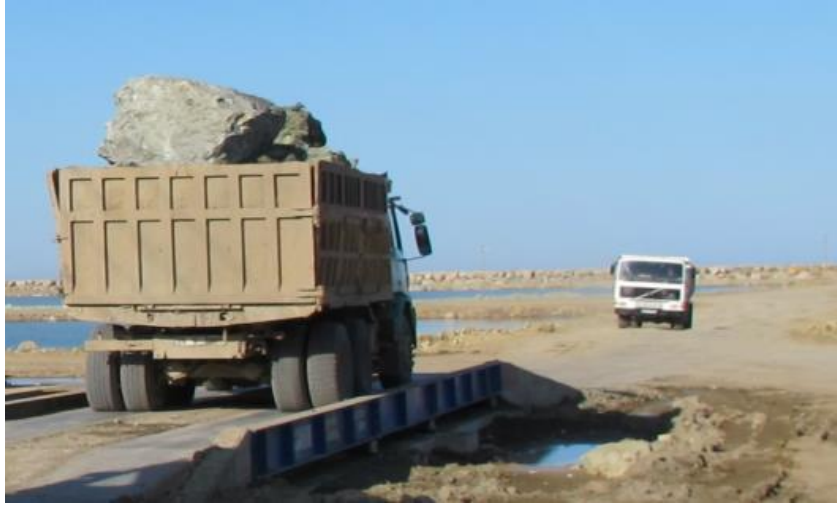
Figure 4.43 Transportation of stones to site by trucks, Retrieved from İbrahim Ahmetođlu, Project Manager of Cengiz Insaat.
