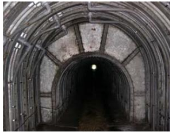
Fig. 10 (a) (b) gallery with a smaller cross sectional layout (width×height=2.07 m×2.1 m) for drainage (c) water-collection chamber with enlarged cross section (width×height=3 m×3 m) and sub-vertical drainage boreholes (water collection pipes) (d) groundwater collected in chamber (e) outlet of gallery
