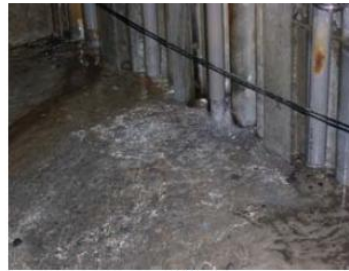
Fig. 10 (a) (b) gallery with a smaller cross sectional layout (width×height=2.07 m×2.1 m) for drainage (c) water-collection chamber with enlarged cross section (width×height=3 m×3 m) and sub-vertical drainage boreholes (water collection pipes) (d) groundwater collected in chamber (e) outlet of gallery
