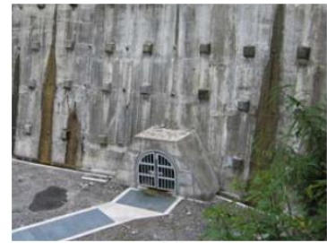
Fig. 10 (a) (b) gallery with a smaller cross sectional layout (width×height=2.07 m×2.1 m) for drainage (c) water-collection chamber with enlarged cross section (width×height=3 m×3 m) and sub-vertical drainage boreholes (water collection pipes) (d) groundwater collected in chamber (e) outlet of gallery
