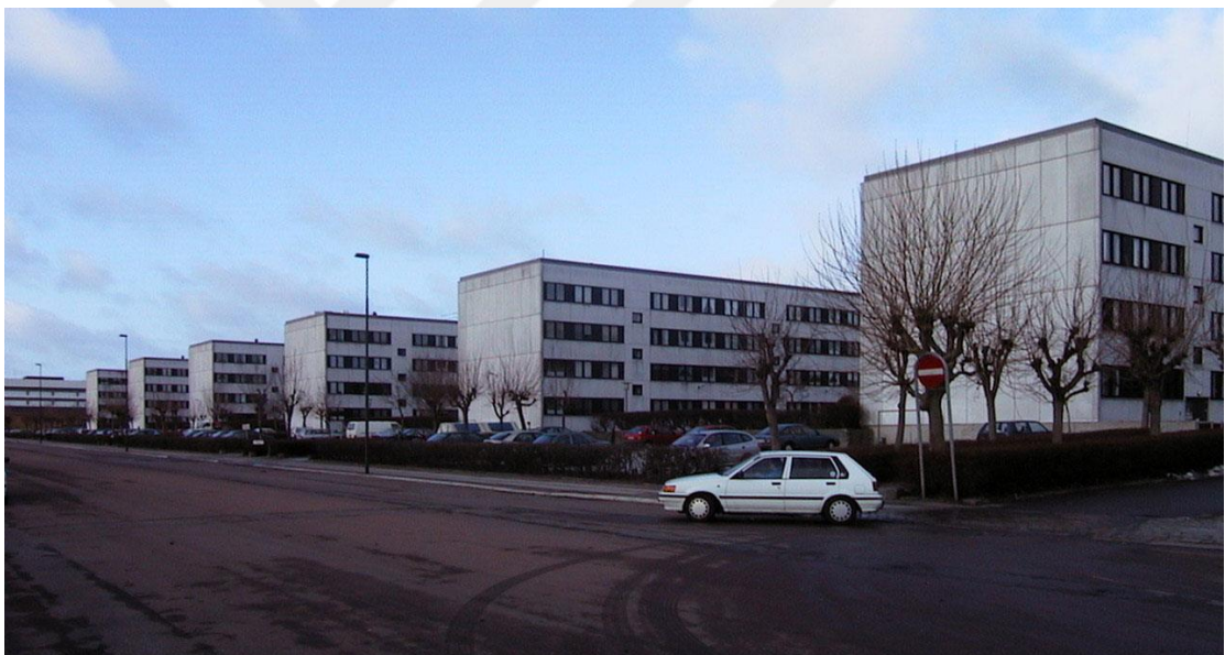
Figure 6-26: Before the renovation. Source: Karen Zwinge Steen/Photoboks
