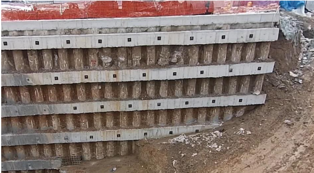
(b) Photograph from the Site
