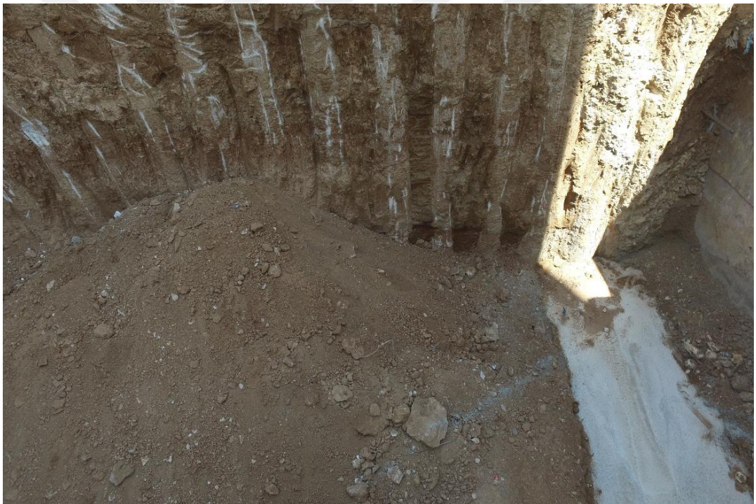
(b) Photograph from the Site
