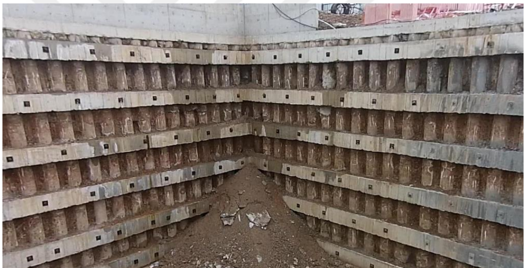
(b) Photograph from the Site
