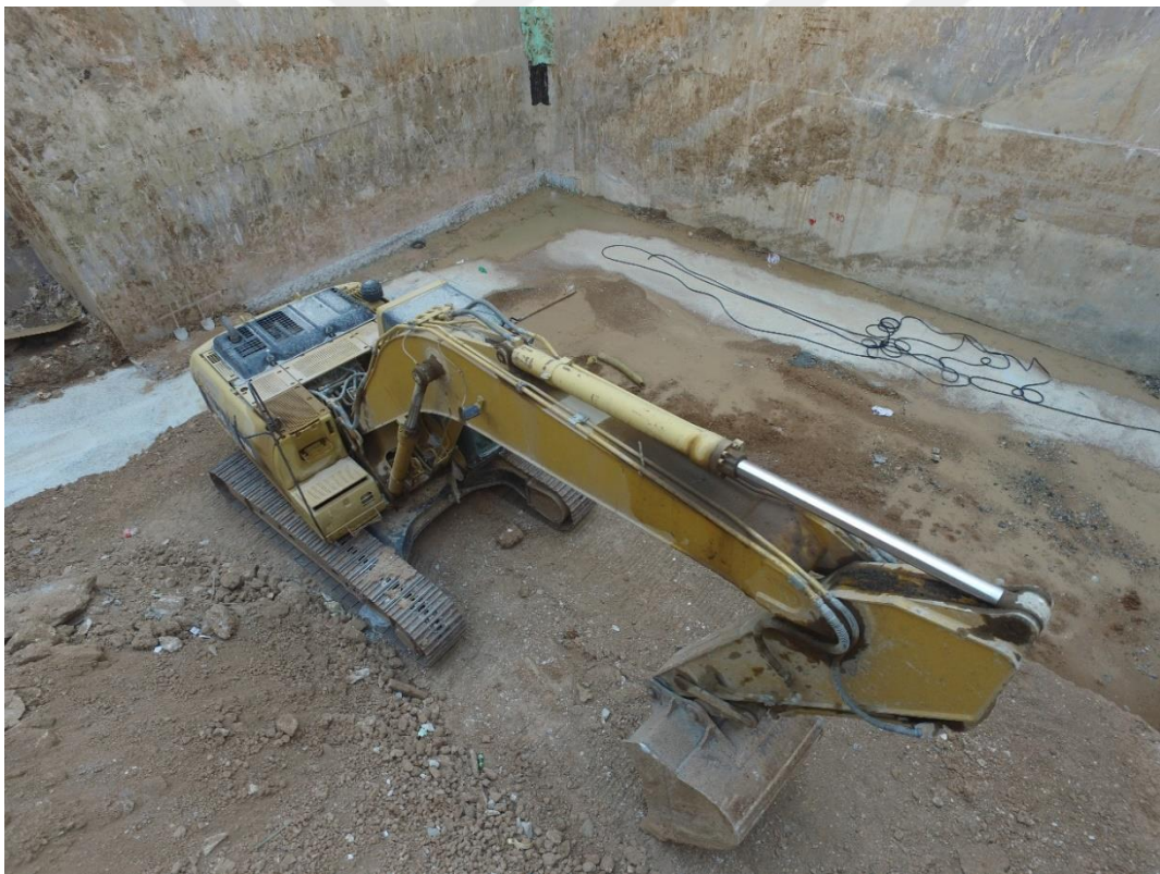
(b) Photograph from the Site
