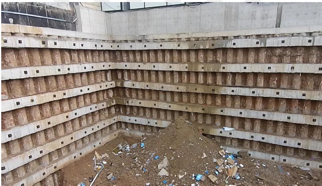
(b) Photograph from the Site
