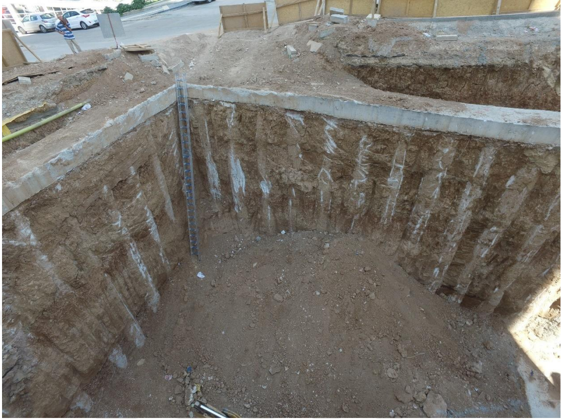
Figure 46 - A Ladder Used to Access the Excavation Site
