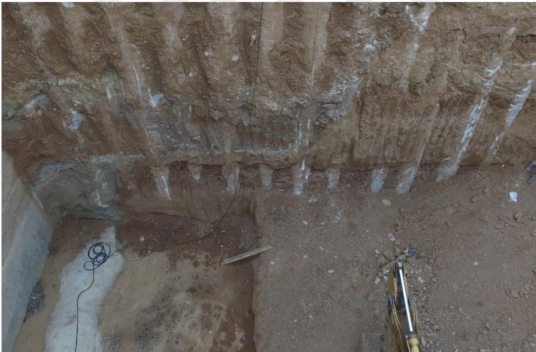
(b) Photograph from the Site
