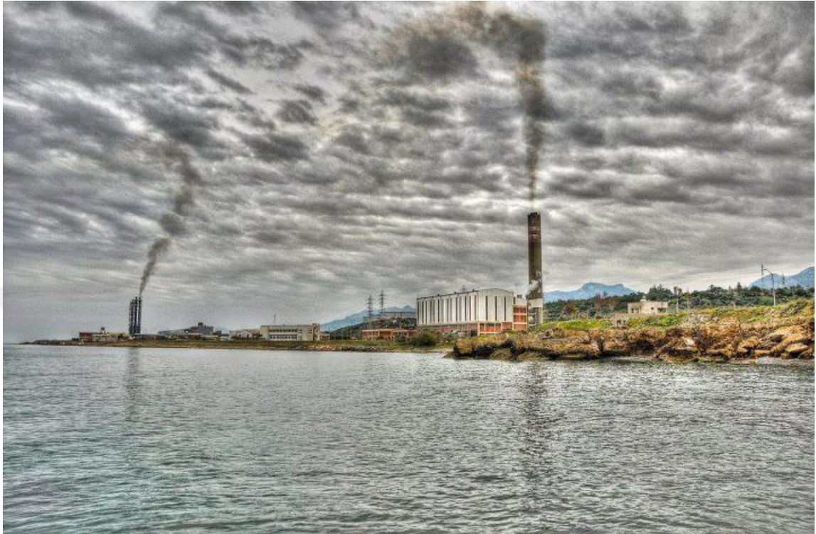
Figure 2: Teknecik Power Plant (Retrieved from: http://www.fotokritik.com/2980184/kktc-teknecik-elektrik-santrali )
