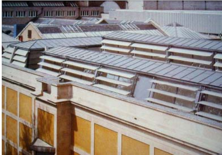
Figure 3.3 : Interior and exterior images from Tate Gallery, London showing the controlled toplighting and solar control system (Wilson M.,2006)
