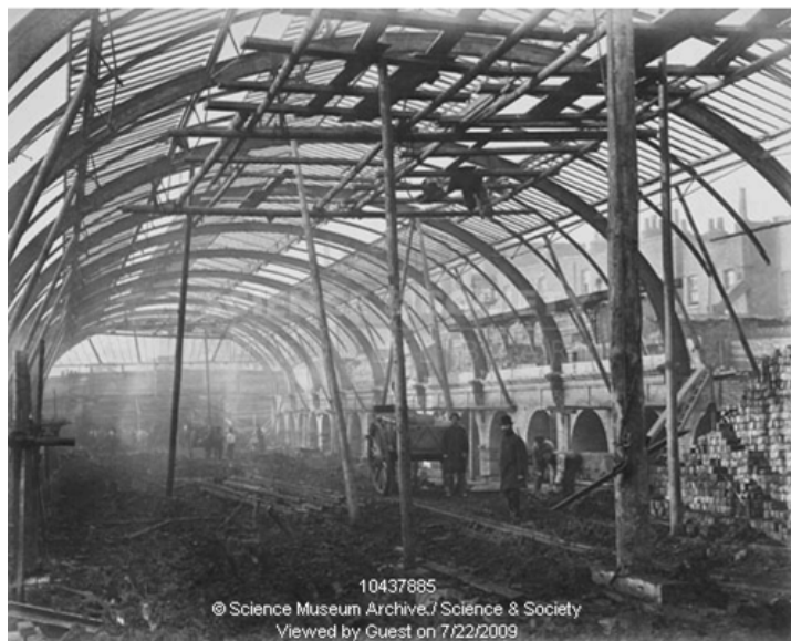
Figure 3.30 Construction of Bayswater Underground Station, 1867
