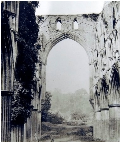
Figure 3.8 Rievaulx Abbey by Francis Bedford, late 1850s
