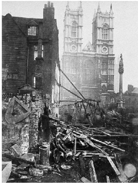
Figure 3.26 Construction of the Metropolitan District Railway, Westminster, 1869
