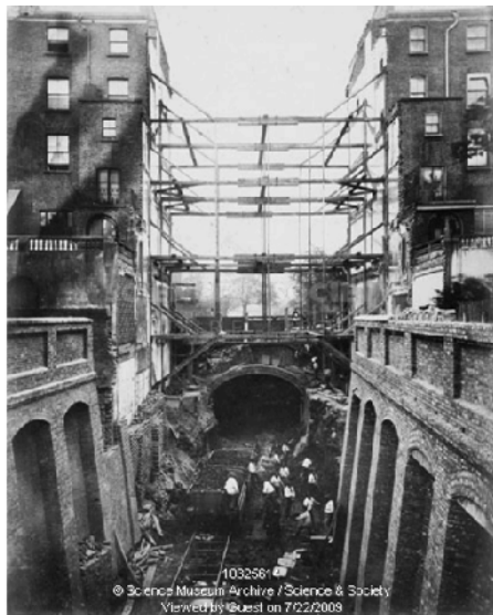
Figure 3.27 Construction of the Metropolitan District Railway, Bayswater, 1867
