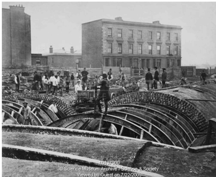
Figure 3.29 Site construction of the Victoria Street, Blackfriars, 1869
