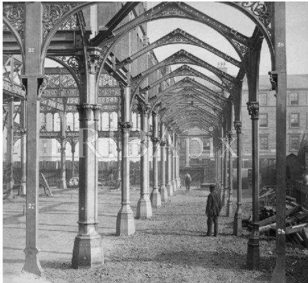
Figure 3.38 Central Market, Santiago: view of the prefabricated structure being assembled in Britain before shipment to Chile, 1860s
