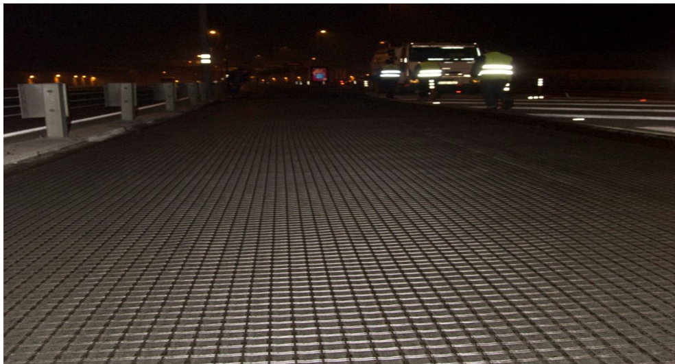
Figure 7.5. Geosynthetic application on METROBUS Line
