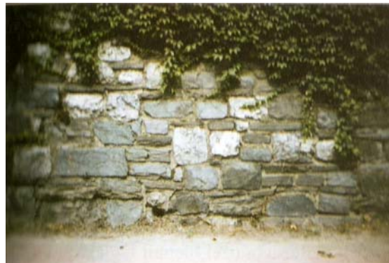
Fig 2.3 : Photograph of a rubble stone wall
