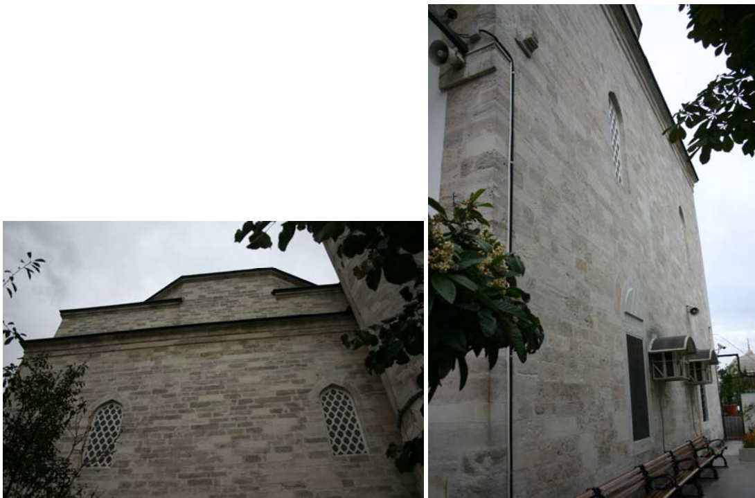
Fig 4.4 : Example of Early Ottoman cut stone wall constructions, Firuzağa Mosque
