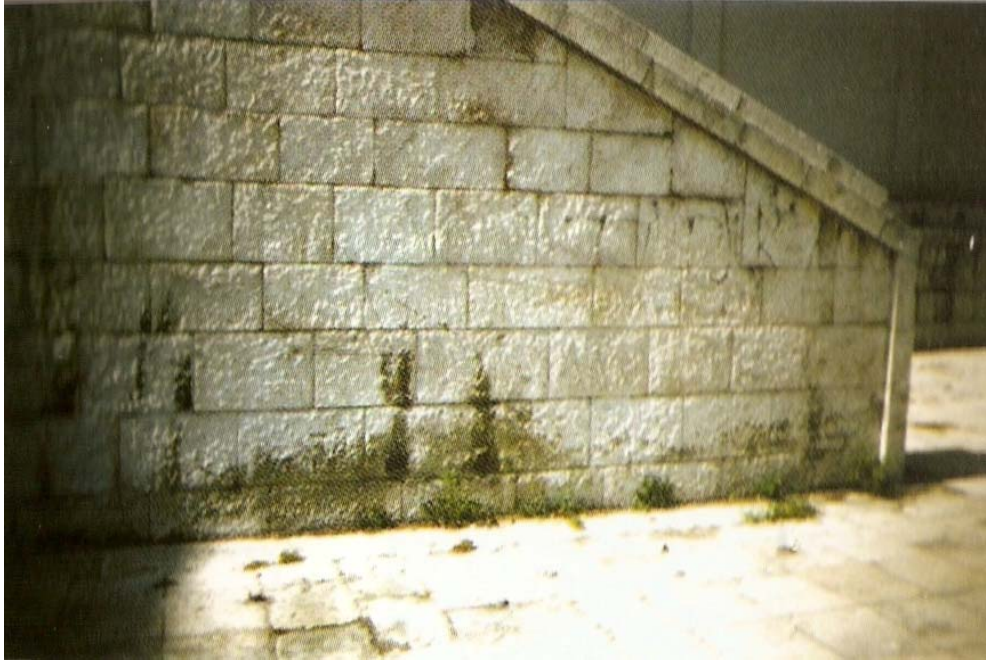
Fig 2.7 : Photograph of a cut stone wall
