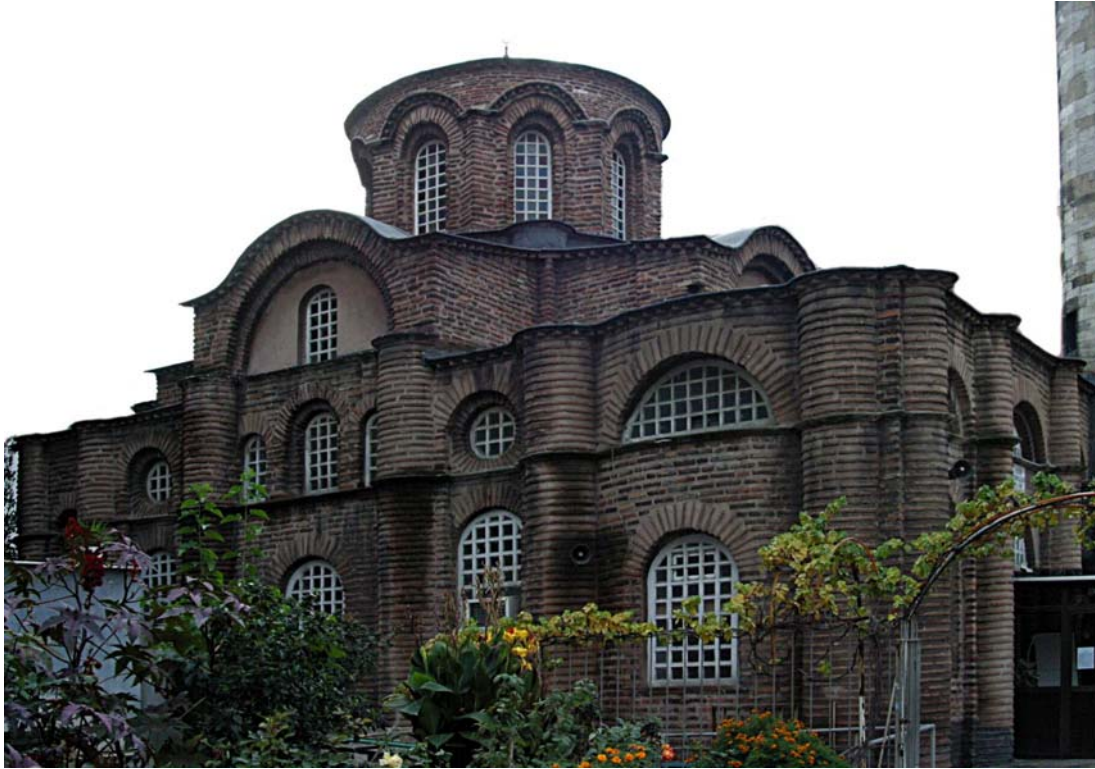
Fig 4.1 : Example of Byzantine brick wall construction, Myreallion Church
