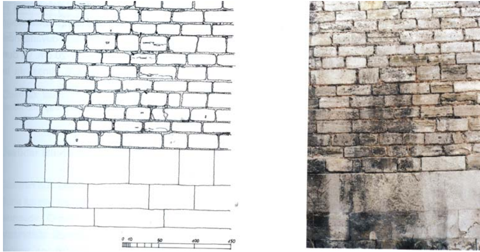
Fig 4.5 : Example of Early Ottoman roughly cut stone wall constructions
